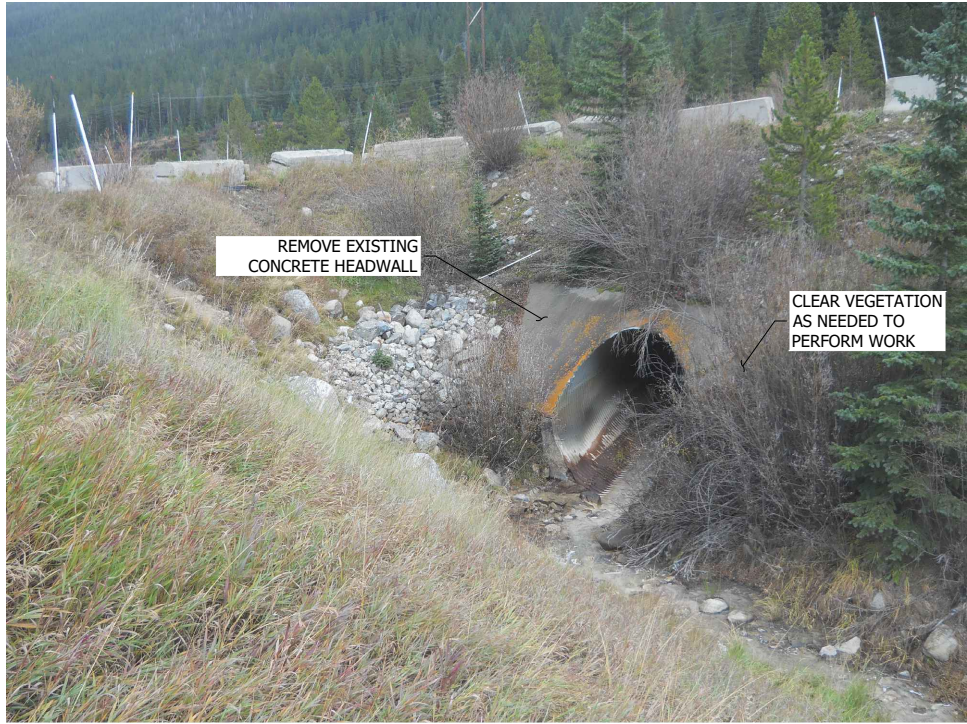
EXISTING CULVERT INLET - 1
