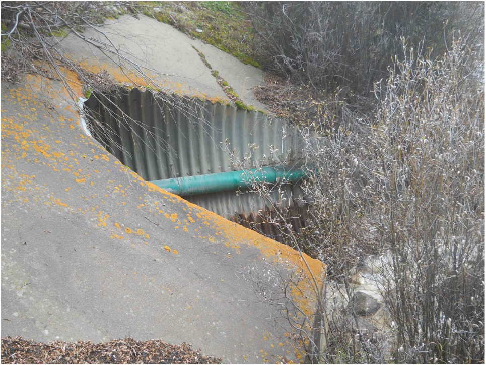
EXISTING CULVERT INLET - 2
