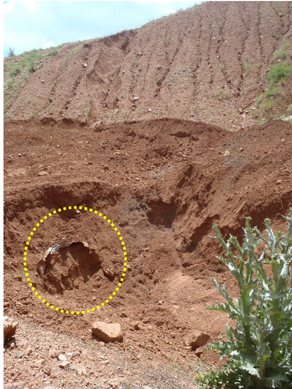
Photo 8. Re-exposed NW culvert inlet (looking SE at area to be regraded, note Scotch thistle lower left).
