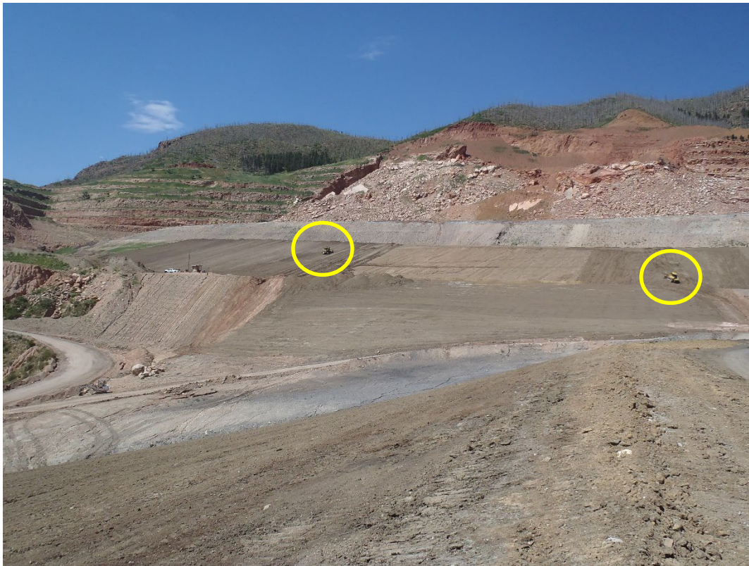
Photo 1. Dozers grading topsoil below lower backfill bench (looking SW).
