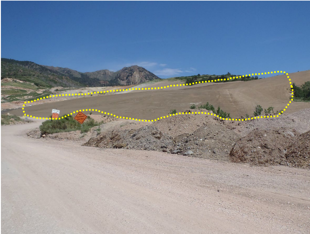
Photo 2. Placed topsoil on regraded former shop area (looking NW).
