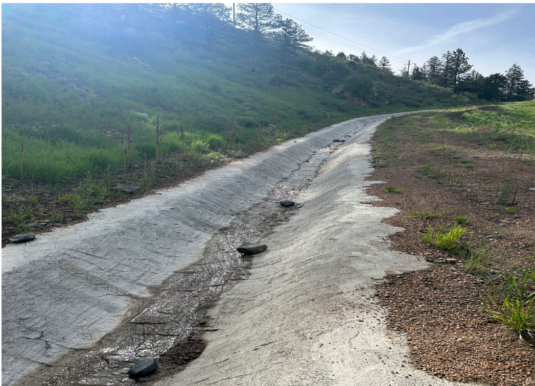
4. Stormwater diversion channel - at north waste rock pile.
