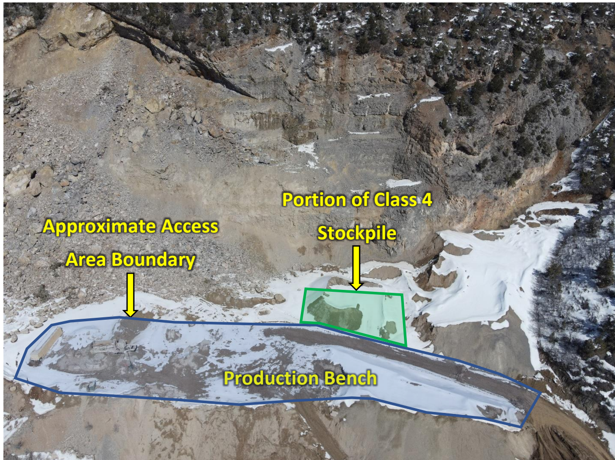
Figure 2 – Production Bench Access Area and Class 4 Stockpile
