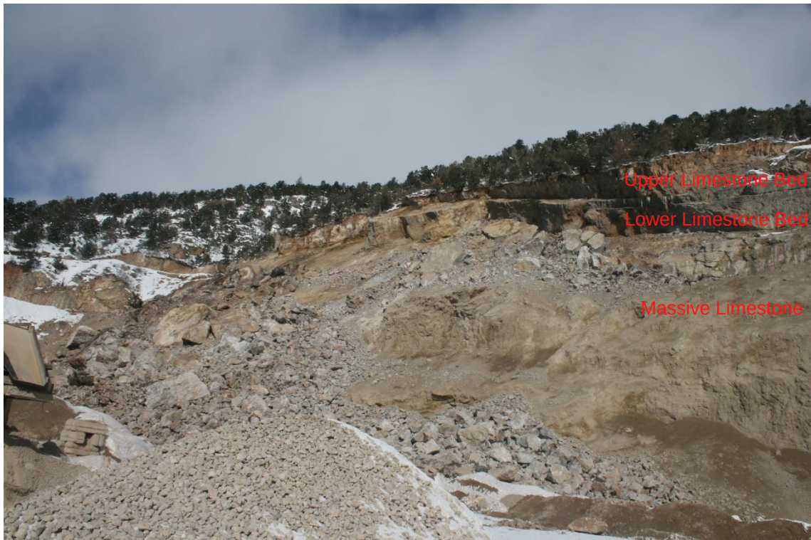
Photo 2: Overview of the January 18, 2023 ground event on the West Face. Rubble path and pile at left. The two upper units of the limestone are visible with bedding acting as the slide plane. (1/26/23 Photo# 0578)
