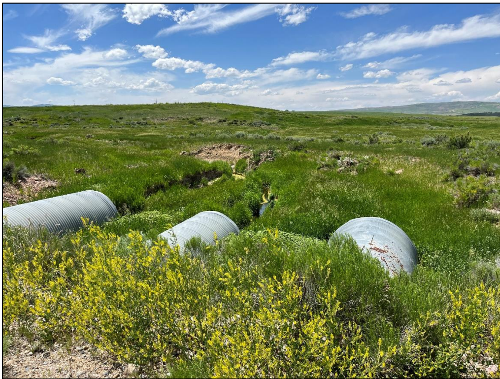
Photo 5: View northwest of culverts which allow Dry Creek to run through the Sage Creek Trail path.
