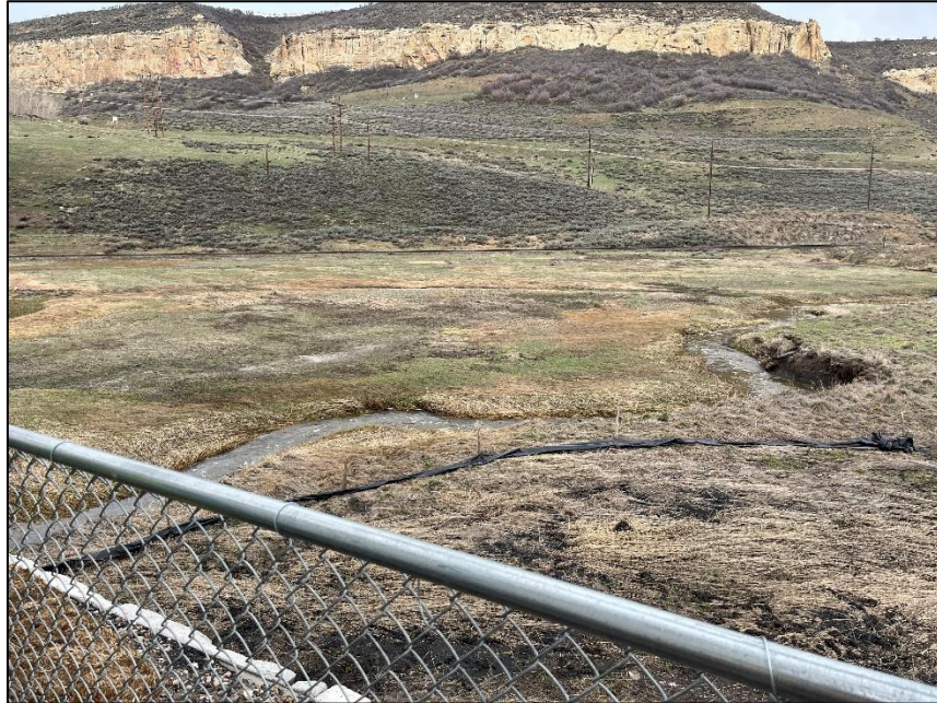
Photo 38: Inspection photo from a previous inspection report dated 5/2/2023 which shows the silt fence behind the stoker loadout building which is in need of repair.
