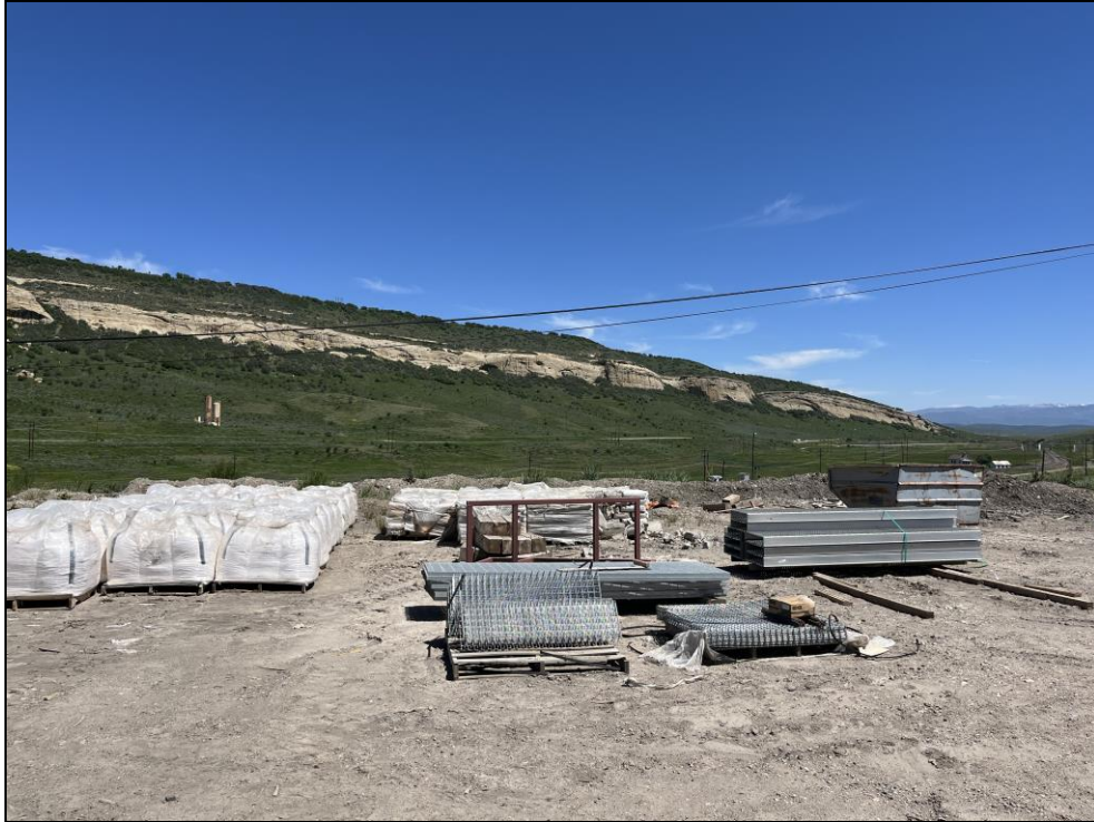
Photo 18: View north of a storage area, berms around this area are being maintained to prevent sediment deposit into the ditch below.
