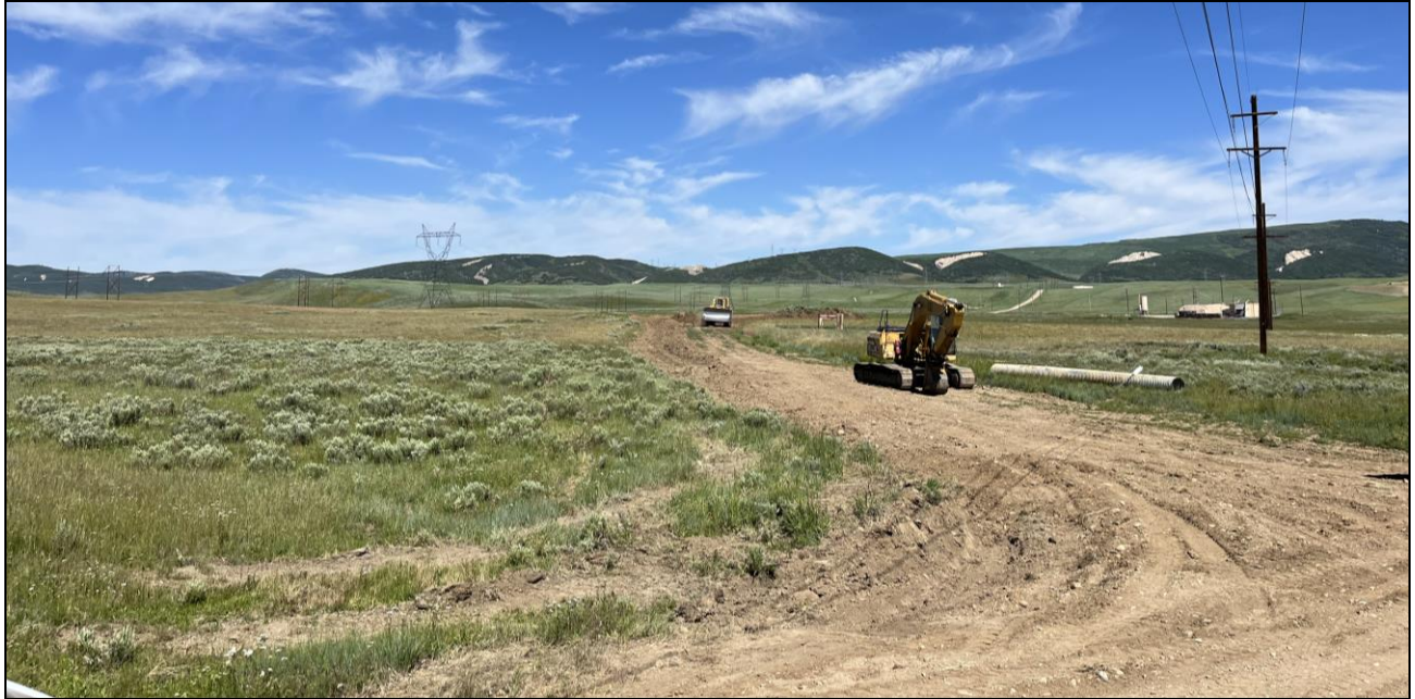
Photo 6: 13 Left Outby Gate Road Utility Borehole is nearly fully reclaimed. Photos shows access road being filled in.
