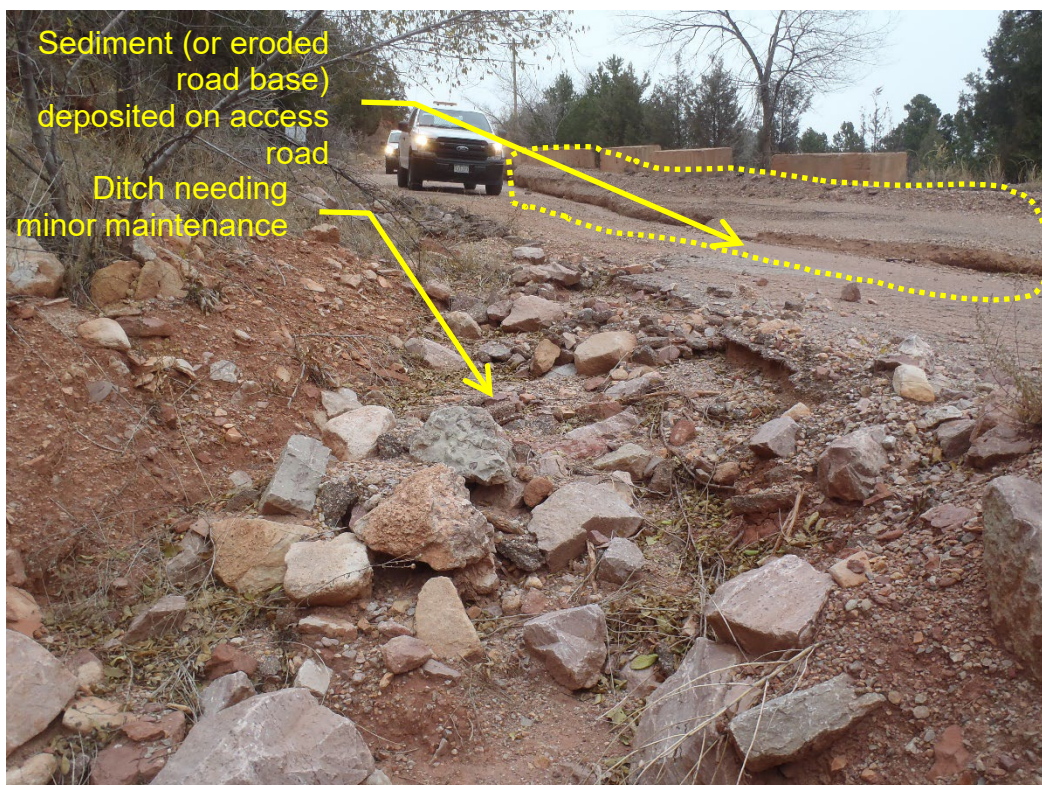
Photo 4. Access road and ditch needing maintenance (looking NW).
