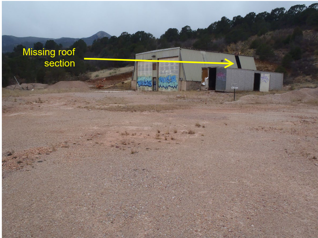
Photo 7. Shop building subjected to vandalism and weather damage.
