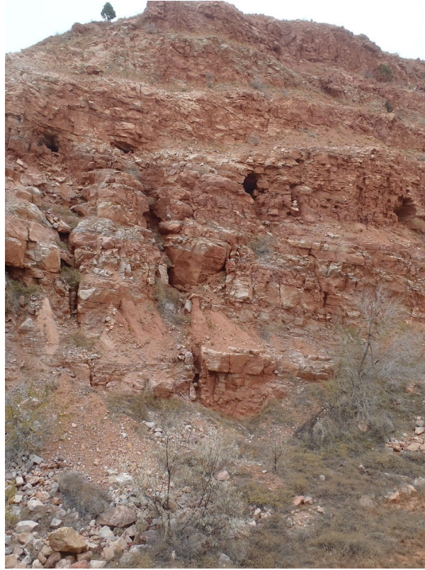
Photo 1. Typical unreclaimed highwall needing scaling, at a minimum (North Phase WP pit, looking NW).
