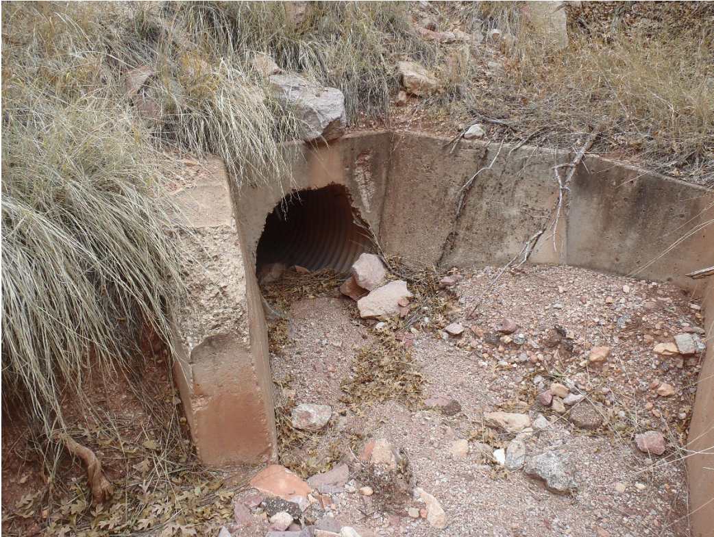
Photo 5. Access road culvert beginning to accumulate sediment (west/inlet side).
