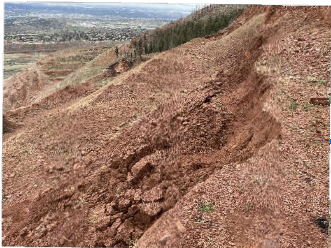
5. Sloughing along upper haul road following rain.
