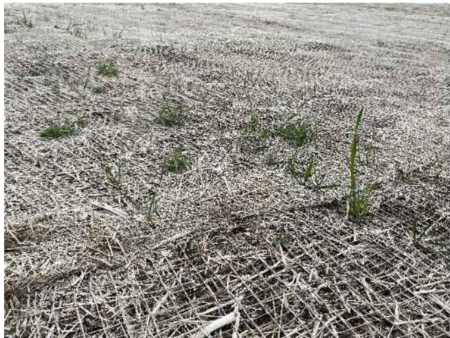
7. Vegetation growing within erosion blanket.
