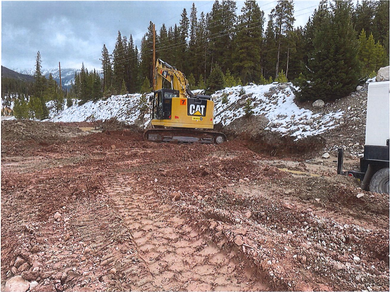
[Photo 4 – Gravel was used to bed pipe and surround the new French drainpipe, then excavation was backfilled]
