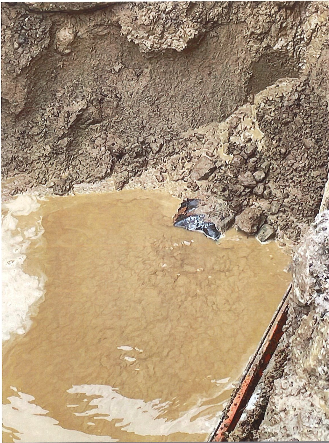
[Photo 1 – Old iron French drainpipe, discovered by following the water that was surfacing by excavating approximately 5 feet down]
