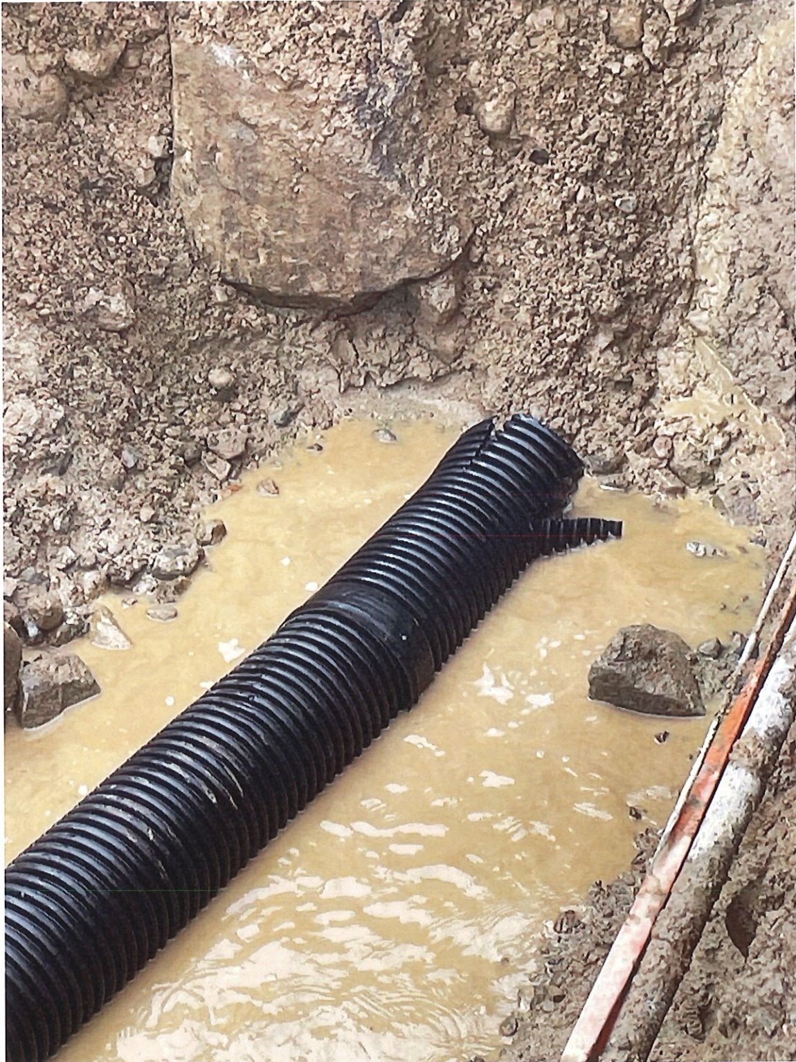
[Photo 2 – New corrugated pipe attached to old French drainpipe]
