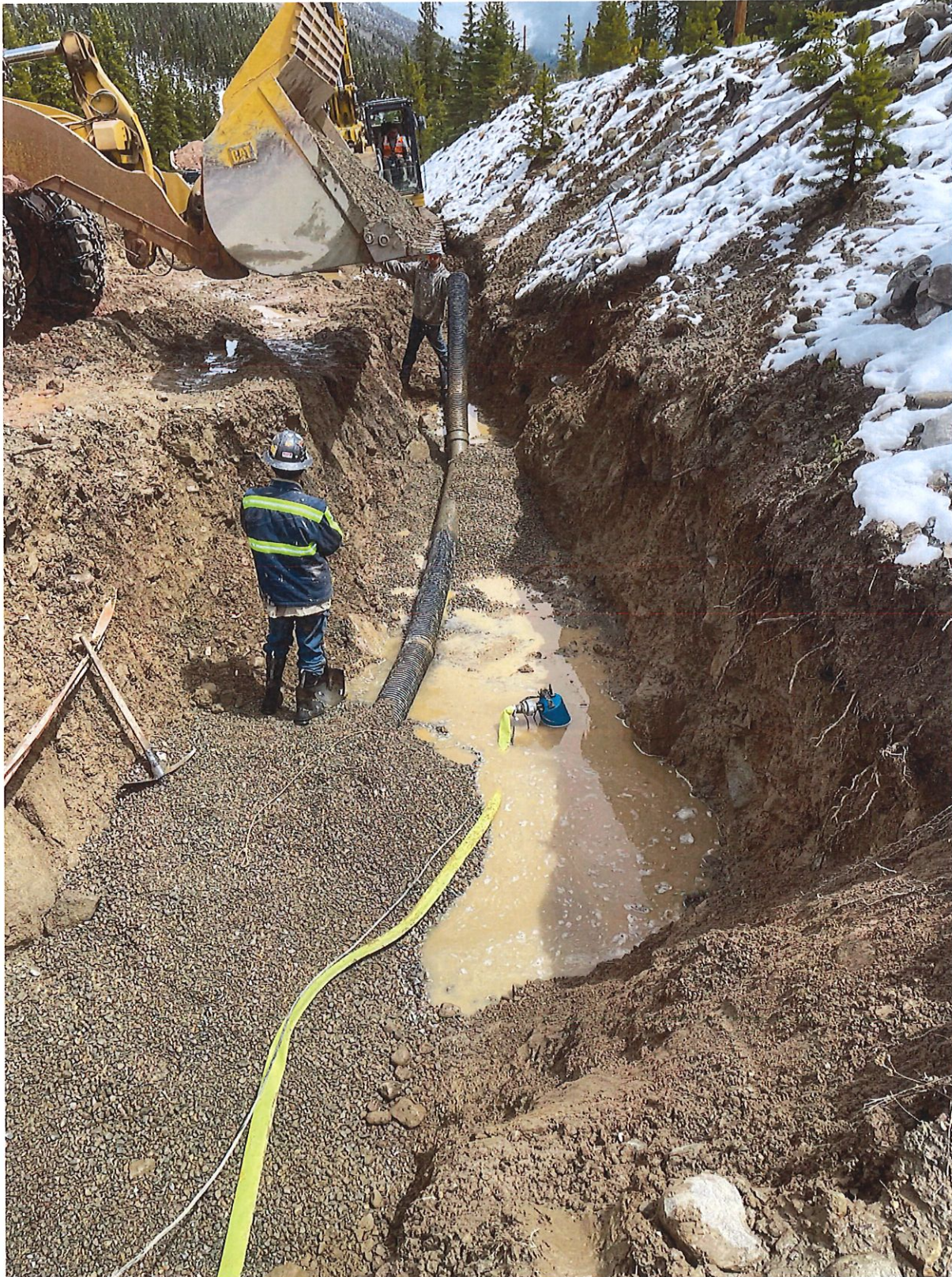
[Photo 3 – New corrugated pipe stretch installed to convey water into existing ditch alongside road]
