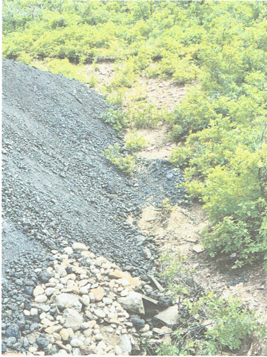
Pic. 5-South side of main waste pile surface runoff point, no erosion protection.
