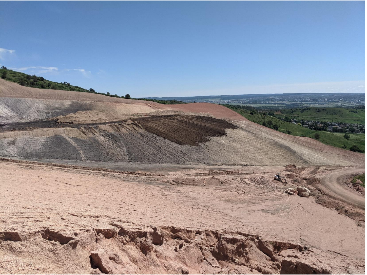
Topsoil placement along north-eastern regraded slope.
