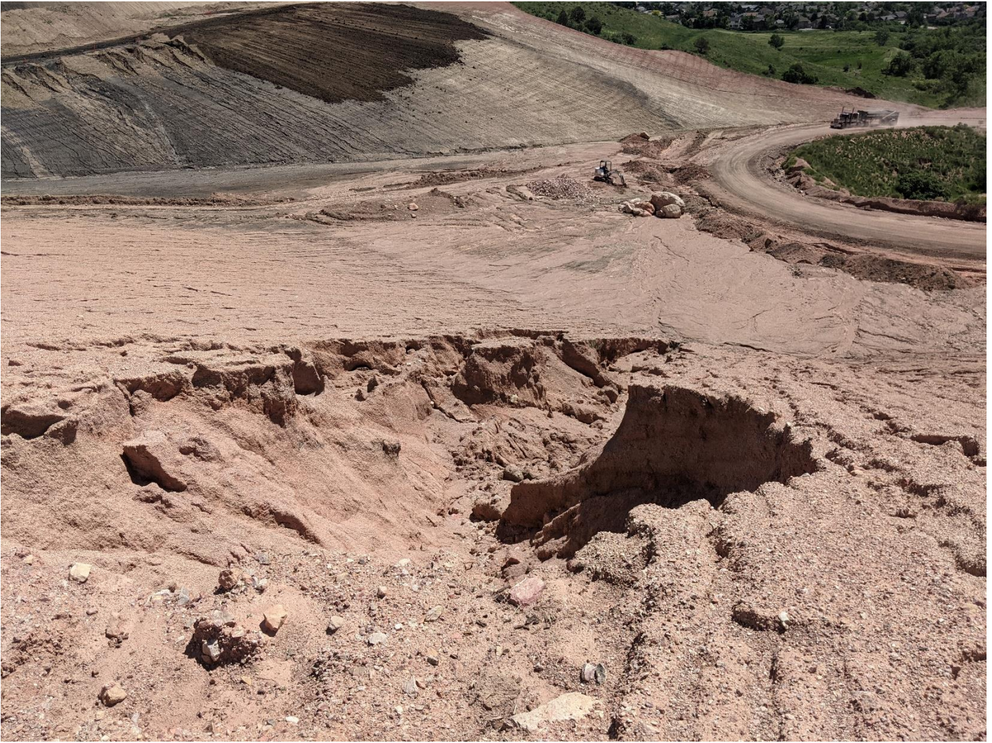
Gully along buttress slope.
