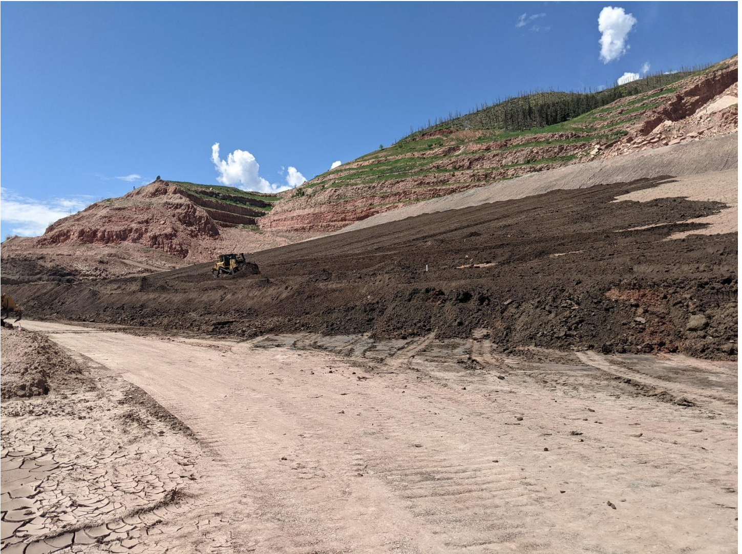
Topsoil placement along the buttress.
