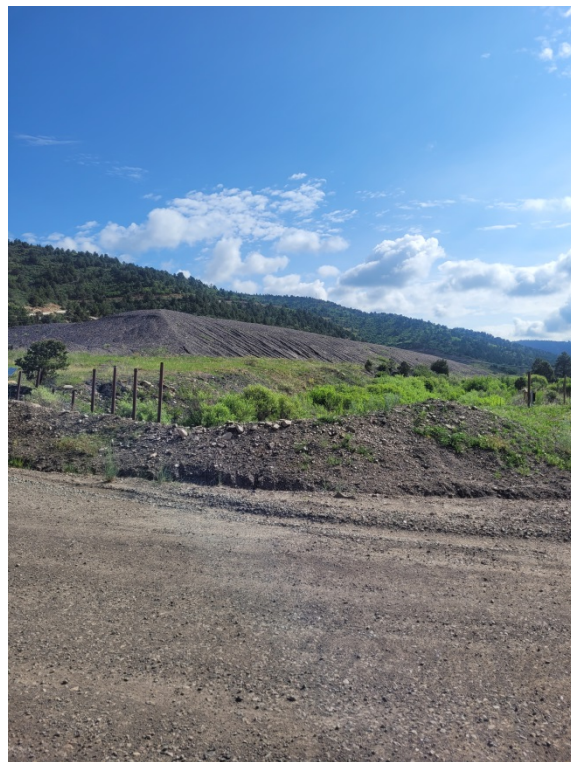
South Facing Side of the DWDA #2
