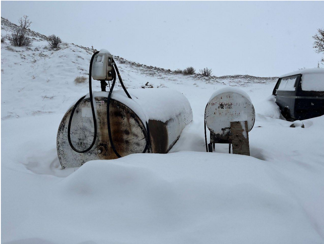
Photo 3: Fuel is stored in secondary containment.
