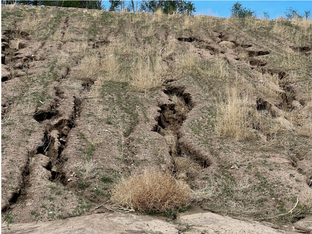
Photo 5. Erosion gullies in central area of buttress in May
