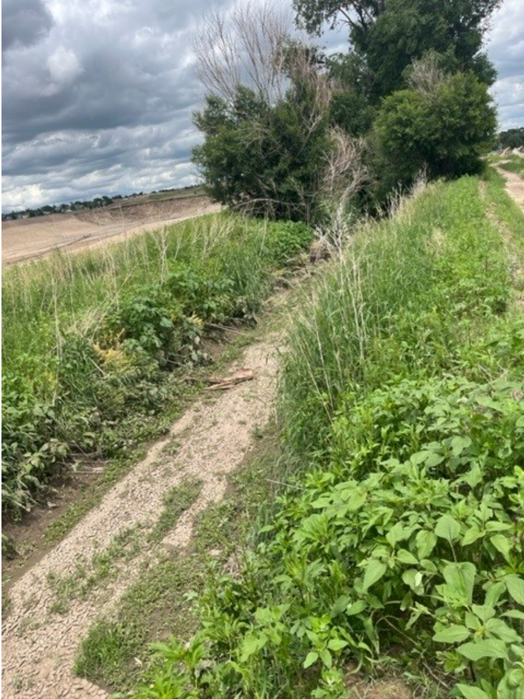
Photo 3. A Dry Fountain Mutual Ditch being separated from the ditch road on right by a berm.
