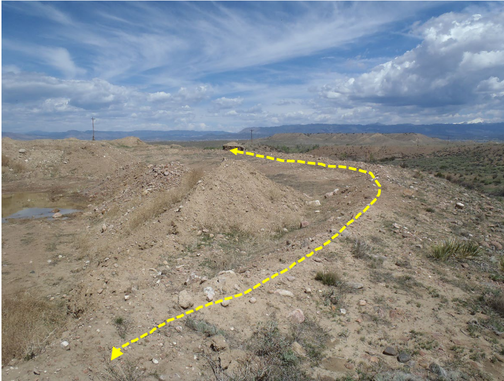
Photo 10. Native material affected area perimeter berm (crest highlighted).
