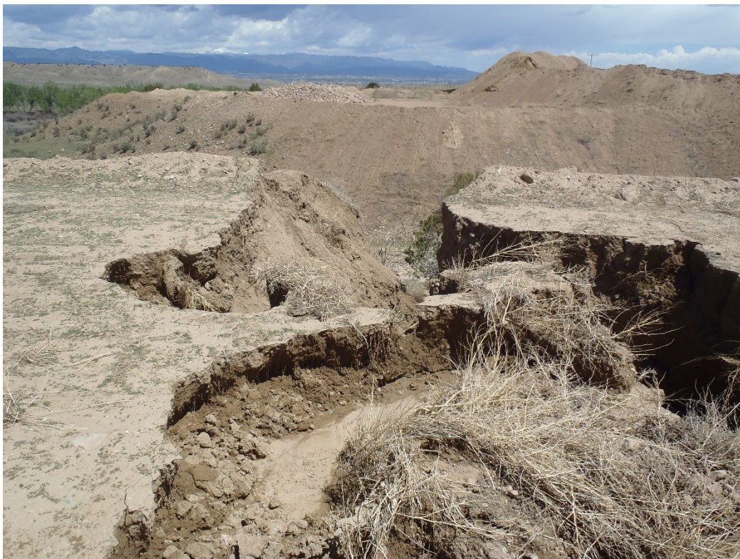
Photo 7. Southwest reclamation area pond erosion gully (looking north).
