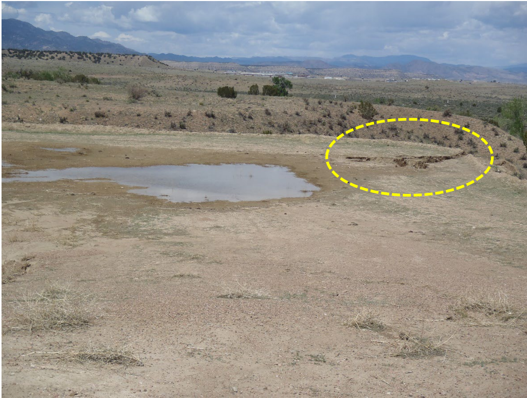
Photo 6. Southwest reclamation area pond – note erosion gully (circled, looking NW).
