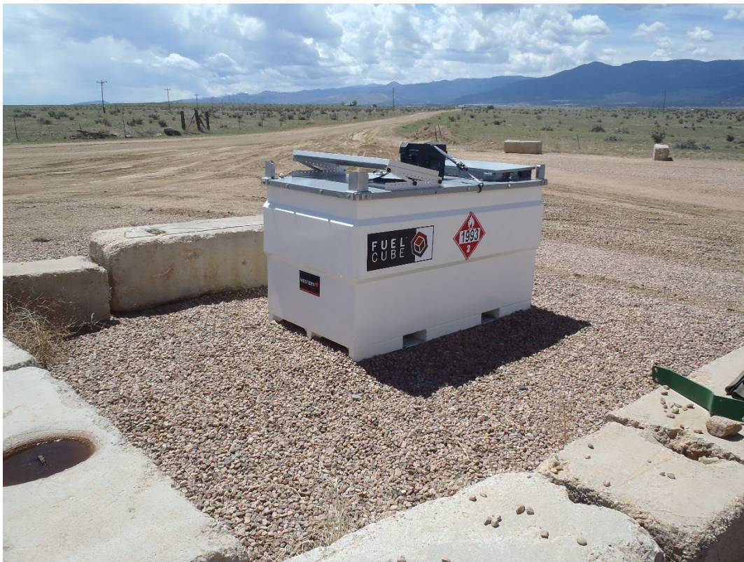
Photo 1. Diesel fuel storage cube (dual walled – near site entrance).
