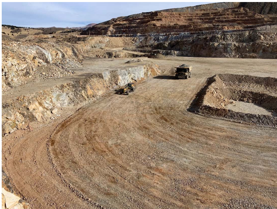
December 5, 2021 – High Compaction Backfill wheel rolling and leveling (TW)
