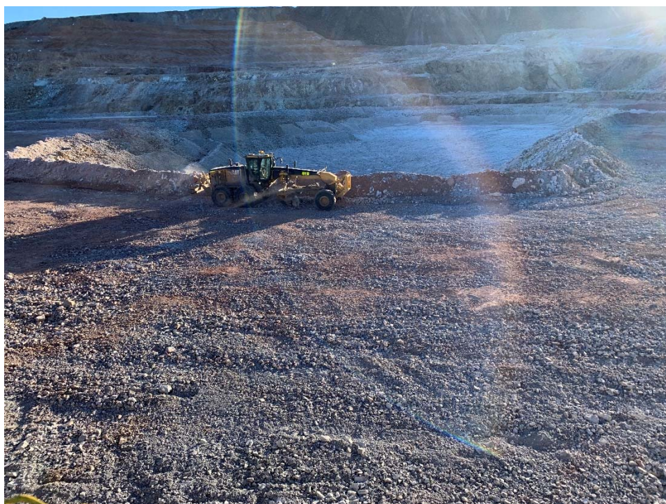
January 21, 2022 – High Compaction Backfill grading (TW)
