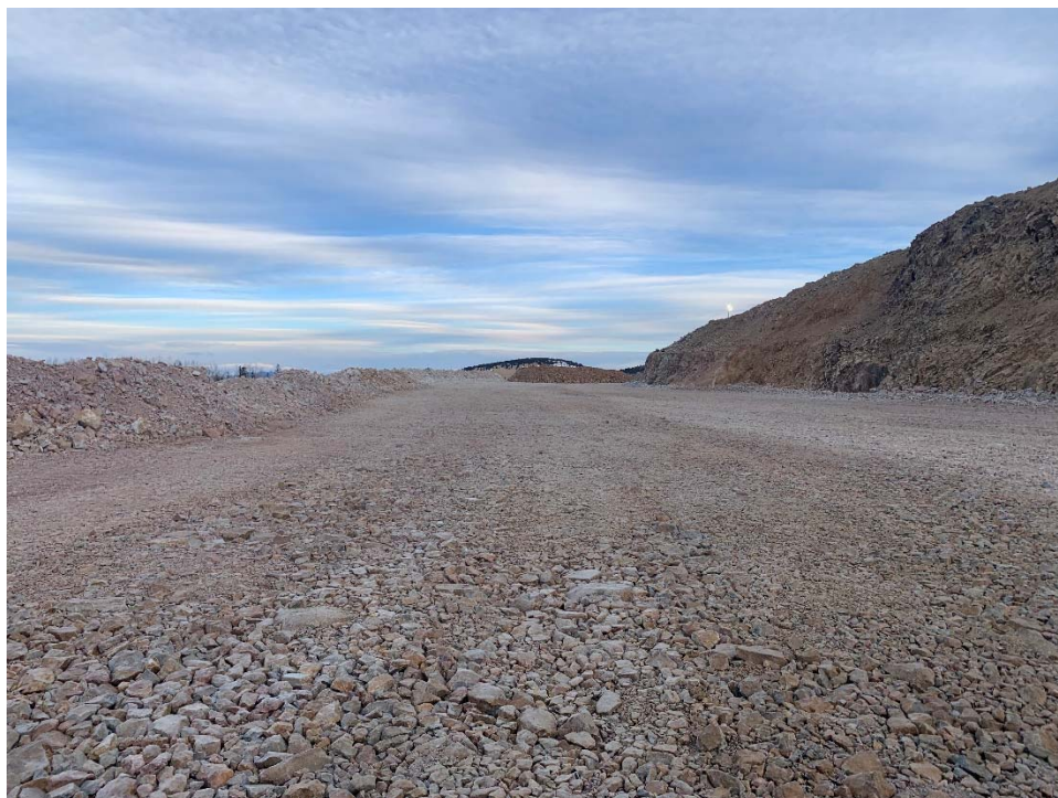
February 21, 2022 – High Compaction Backfill visual inspection (TW)
