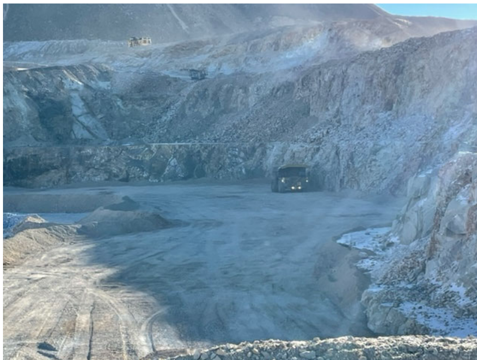
December 30, 2021 – High Compaction Backfill wheel rolling and leveling (GF)
