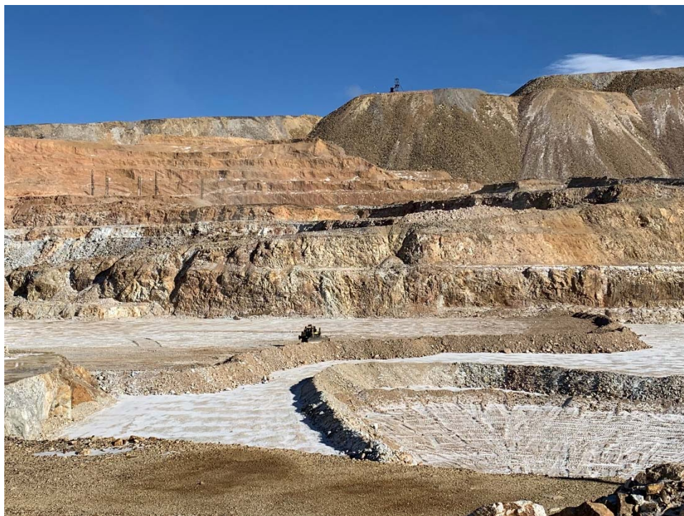
December 16, 2021 – High Compaction Backfill placement (TW)
