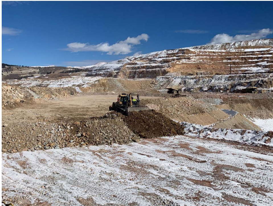
January 24, 2022 – High Compaction Backfill placement (TW)
