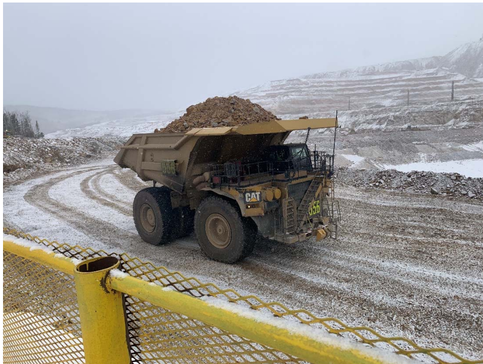
January 25, 2022 – High Compaction Backfill wheel rolling (TW)
