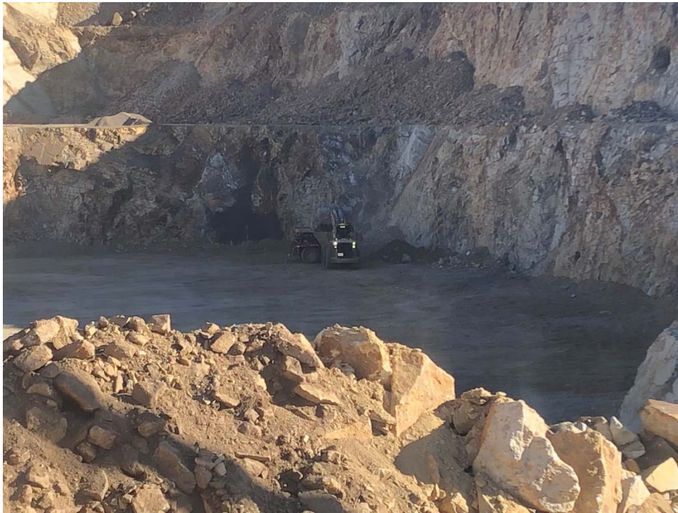
December 1, 2021 – Unsuitable and windrowed material removal (GF)
