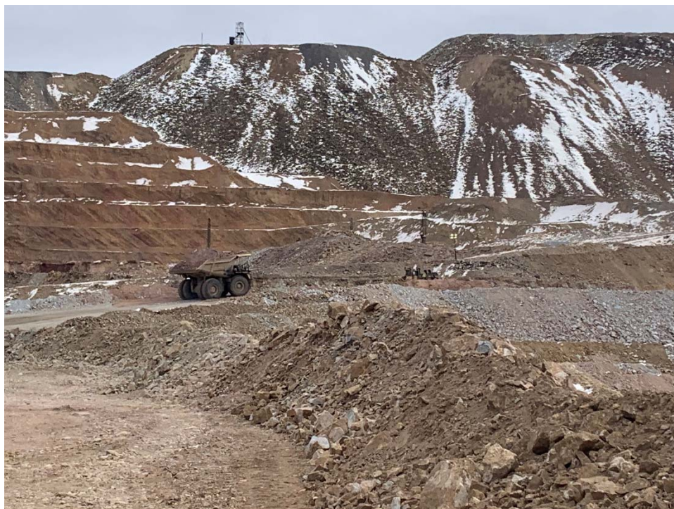
February 21, 2022 – High Compaction Backfill placement (TW)
