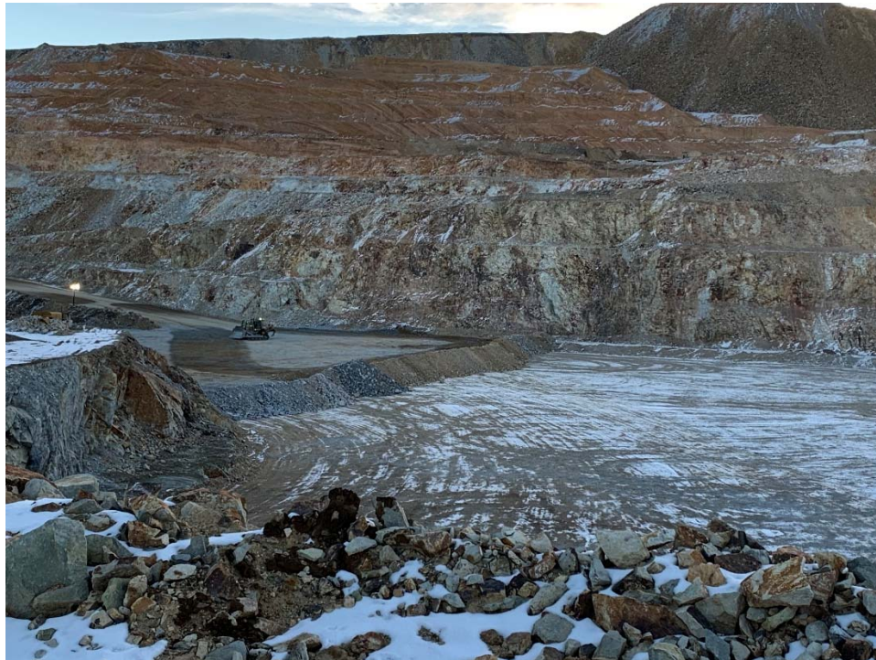
November 22, 2021 – High Compaction Backfill placement (TW)
