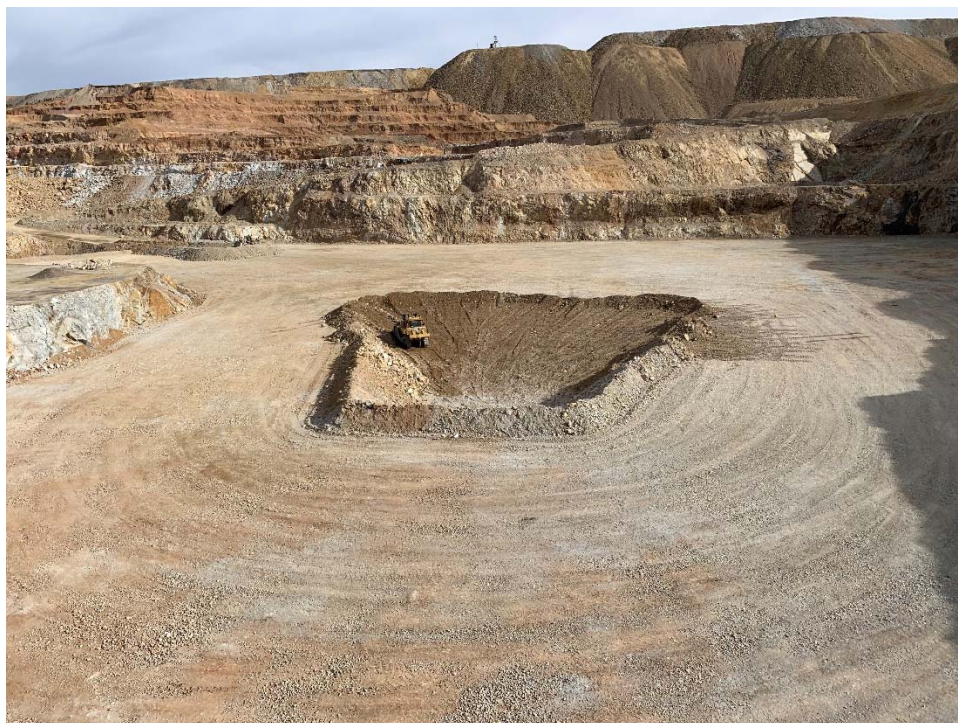
December 1, 2021 – High Compaction Backfill cut contouring (TW)
