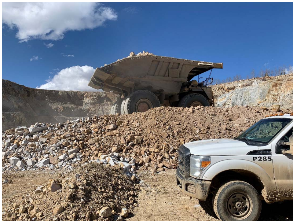
October 18, 2021 – High Compaction Backfill Test Pad wheel rolling progress (TW)
