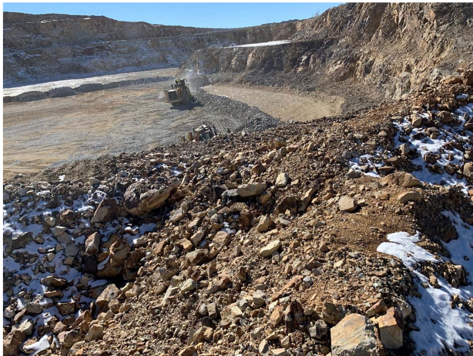
November 22, 2021 – High Compaction Backfill placement (TW)
