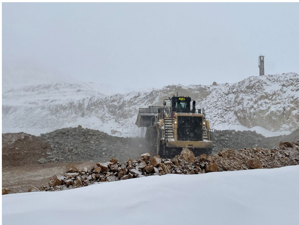
February 2, 2022 – High Compaction Backfill placement (GF)
