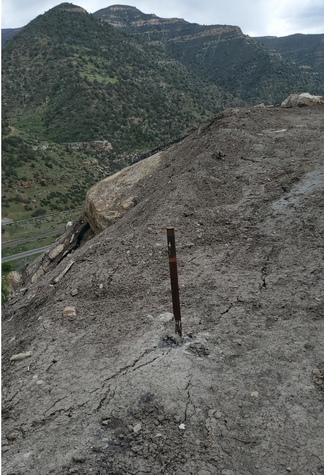
Figure 7: Cracking on benchtop pad (1 of 2)
