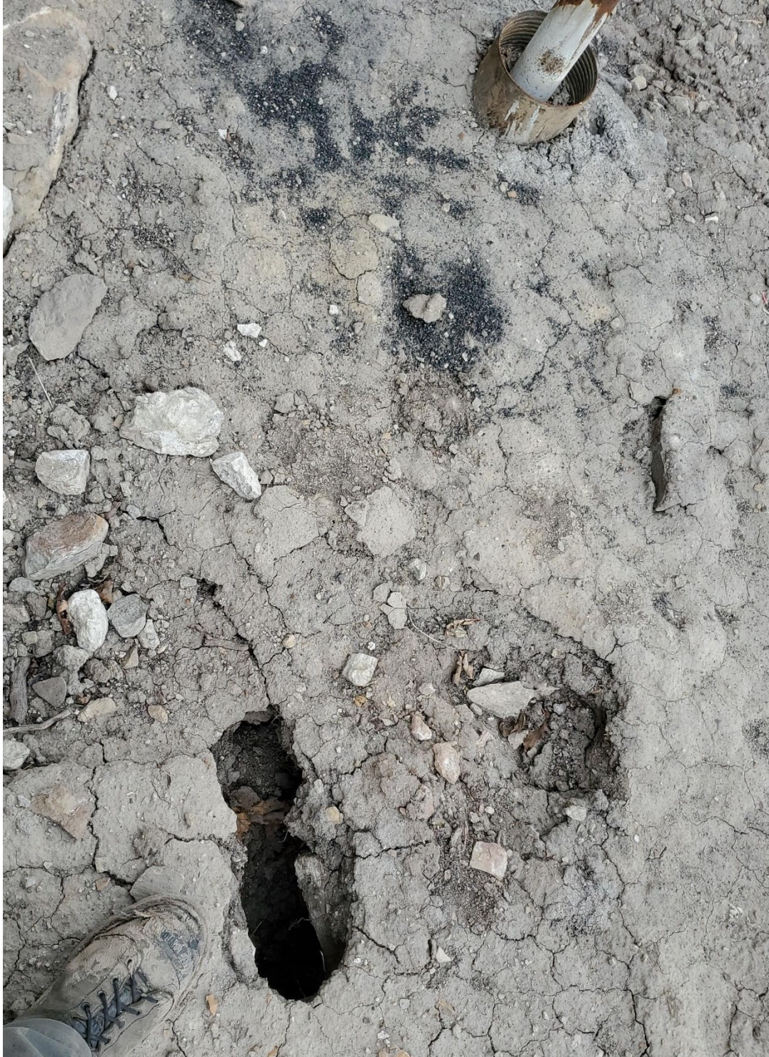
Figure 9: Possible subsidence on benchtop pad
