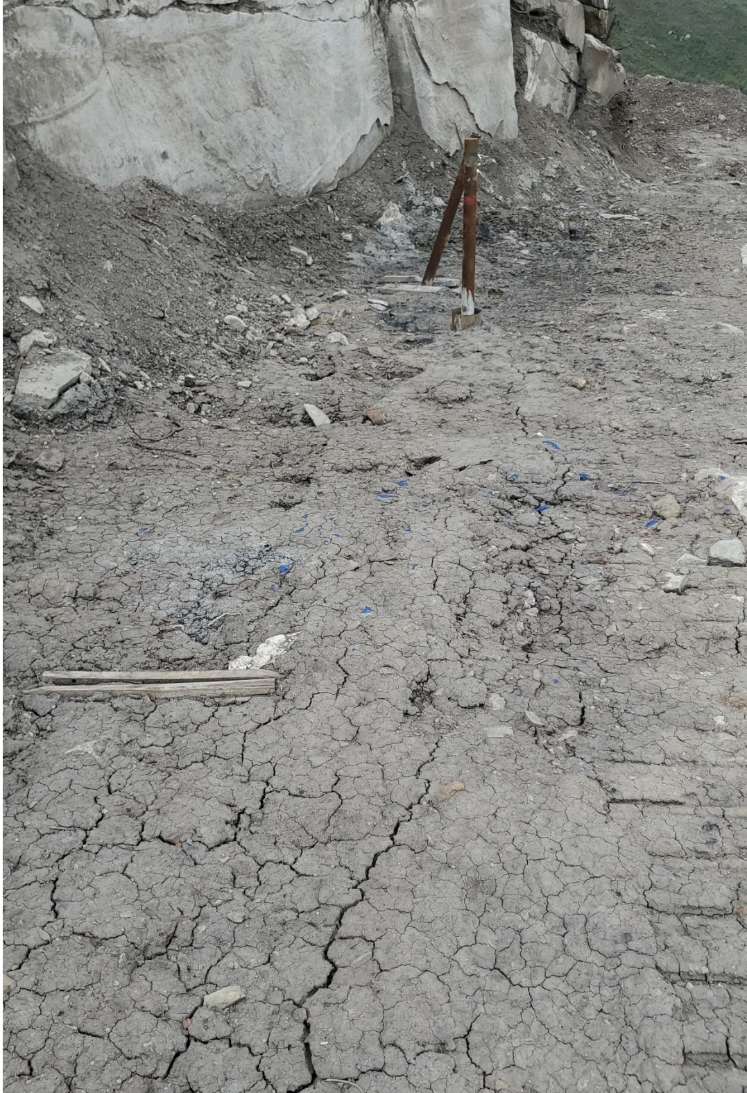
Figure 8: Cracking on benchtop pad (2 of 2)
