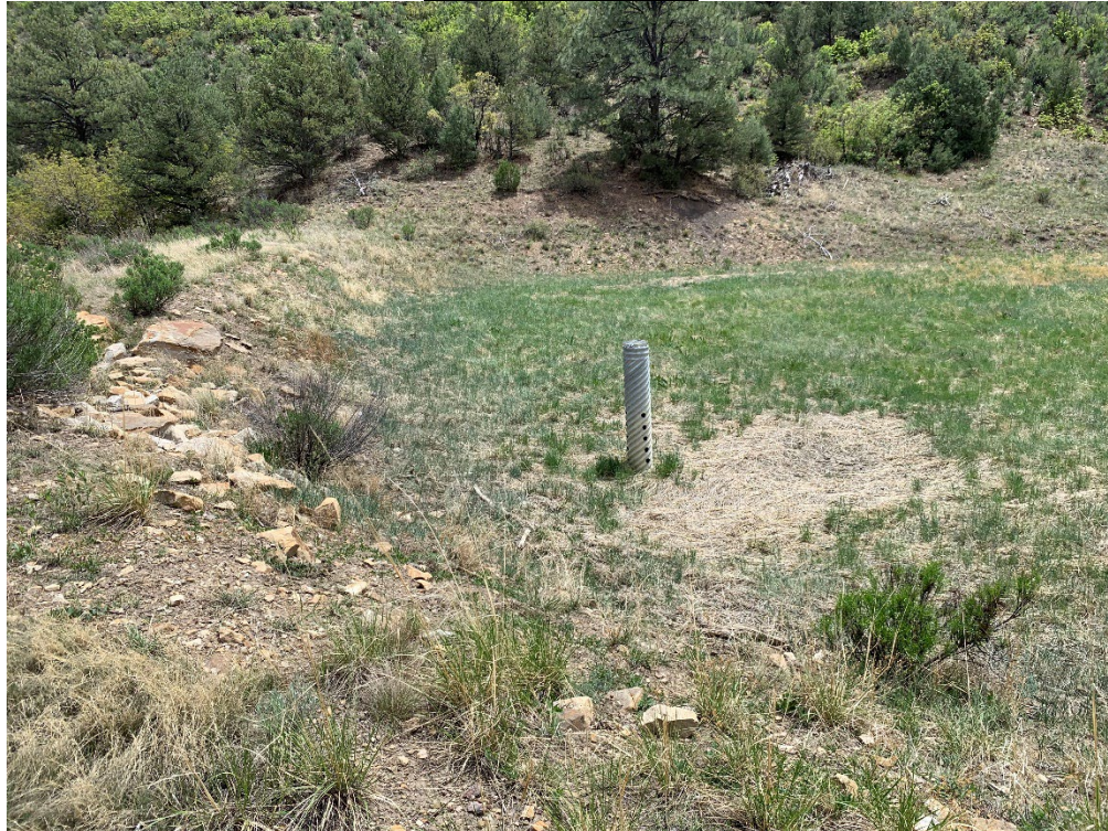
Photo 1 – Pond 5 Primary spillway and embankment
