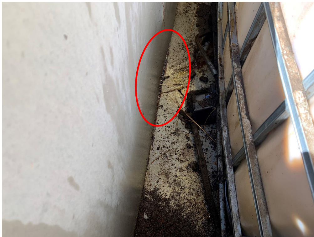
Photo 8 – Break in the secondary containment floor
