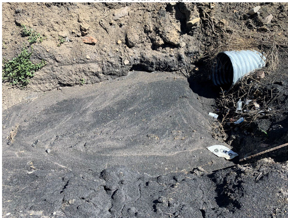
Photo 3 – The sump at culvert C64 needs cleaning
