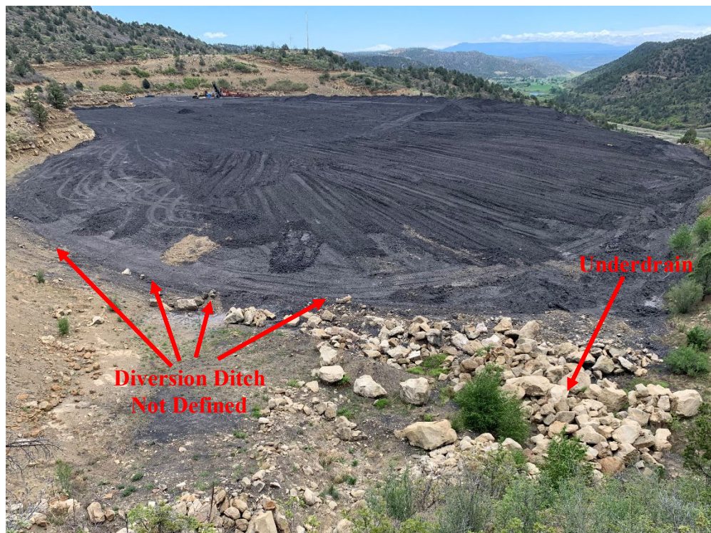
Photo 6 – Perimeter Ditch needs direct water past underdrain
