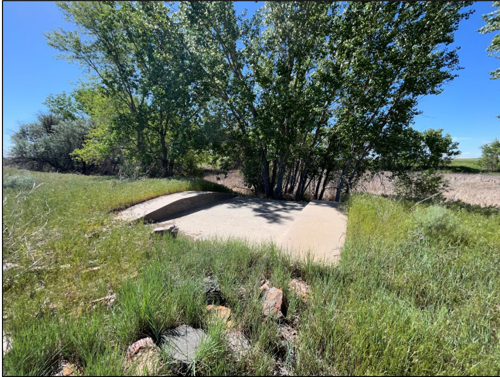
Photo 3: Spillway at Sediment Pond 2
