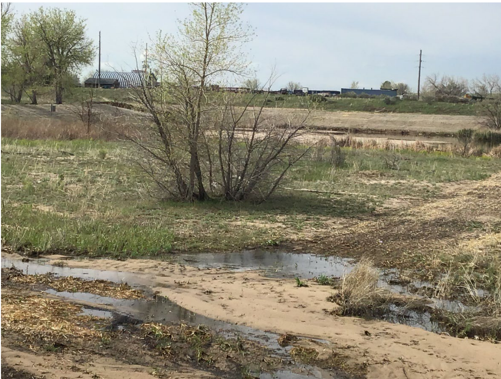
Photo 2. Looking south to eastern section ponds. Banks are blanketed and seeded.
