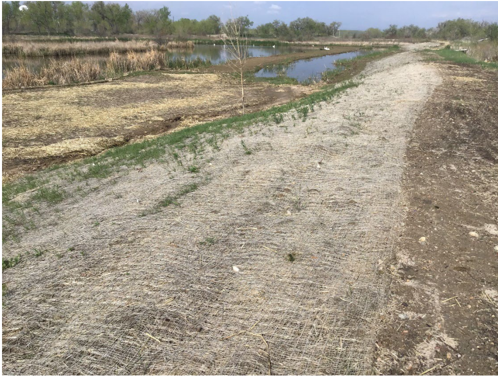
Photo 5: Example of the erosion/ vegetation blankets and the slopes along the ponds.
