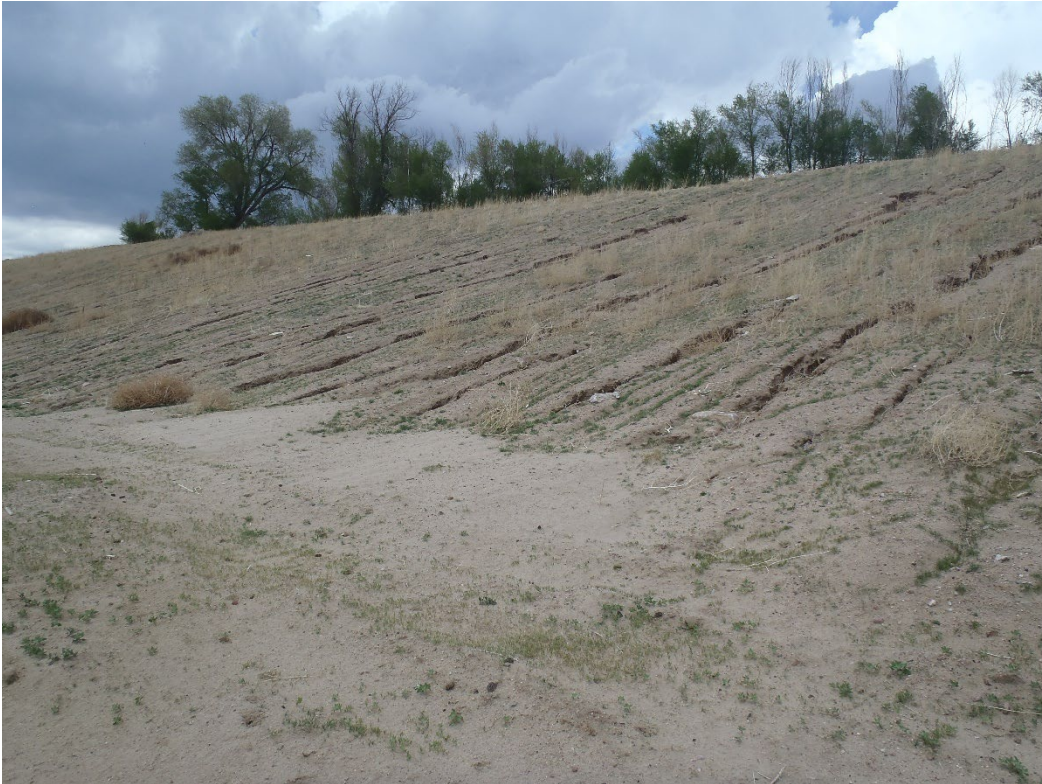
Photo 5. Heavy erosion rilling on west buttress fill (looking NW).
