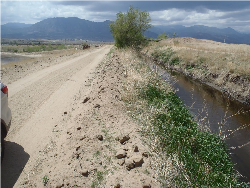
Photo 3. Ditch and access road at crest of buttress fill (looking west, no rill/headcutting at crest on left).
