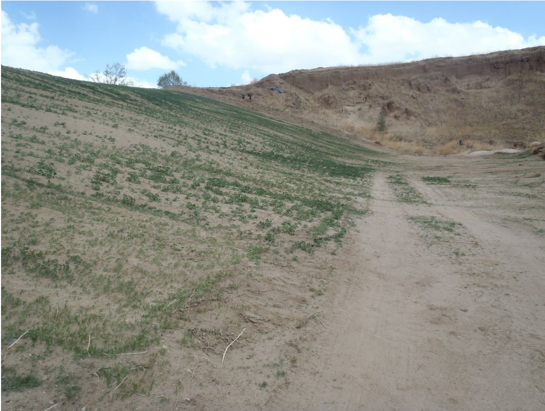
Photo 1. Regraded and hydromulched east end of buttress fill (looking east).
