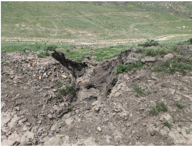
Collection ditch breach.
