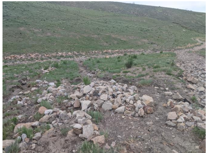
Breached area of East Taylor Ditch.
