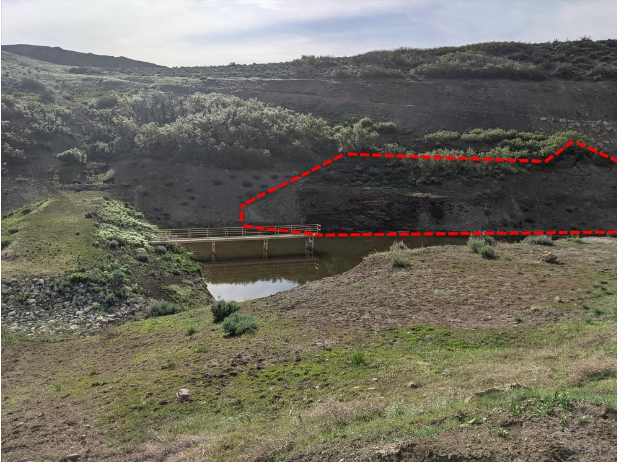
Approximate outline of slump at Section 26 Pond.
