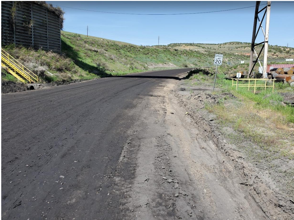
Photo 10: View to the west of haul road. Ditch has been pulled and road was wet from water truck.
