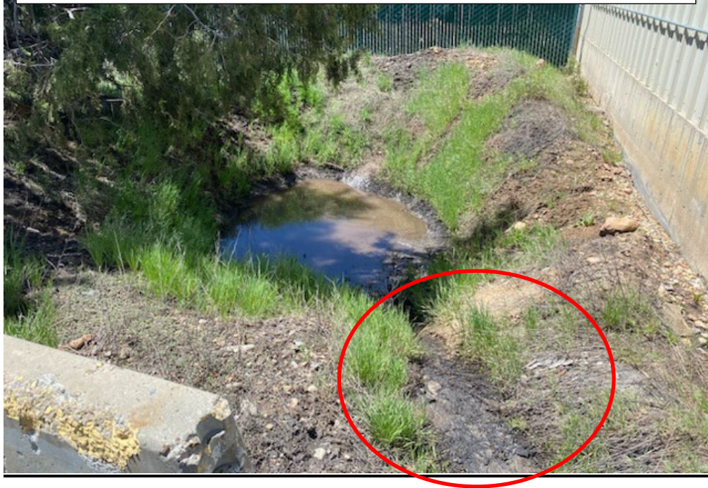
Photo 9: The inlet from the ditch into the sump behind the fuel storage building at the King II Mine
