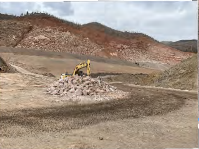
8. Riprap sorted and stored on site for swales and terraces.
