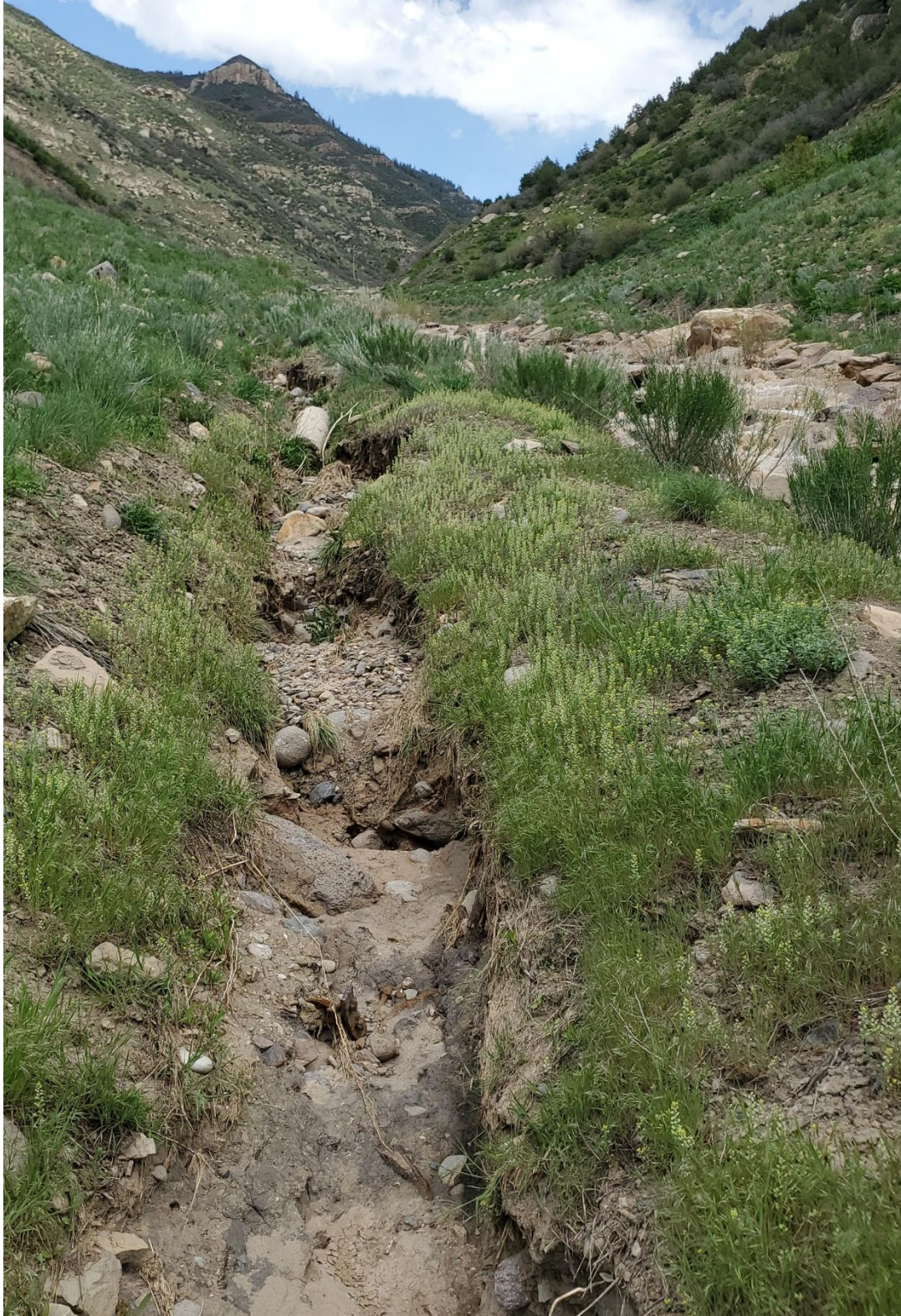
Figure 14: Erosion in Ditch T-1
