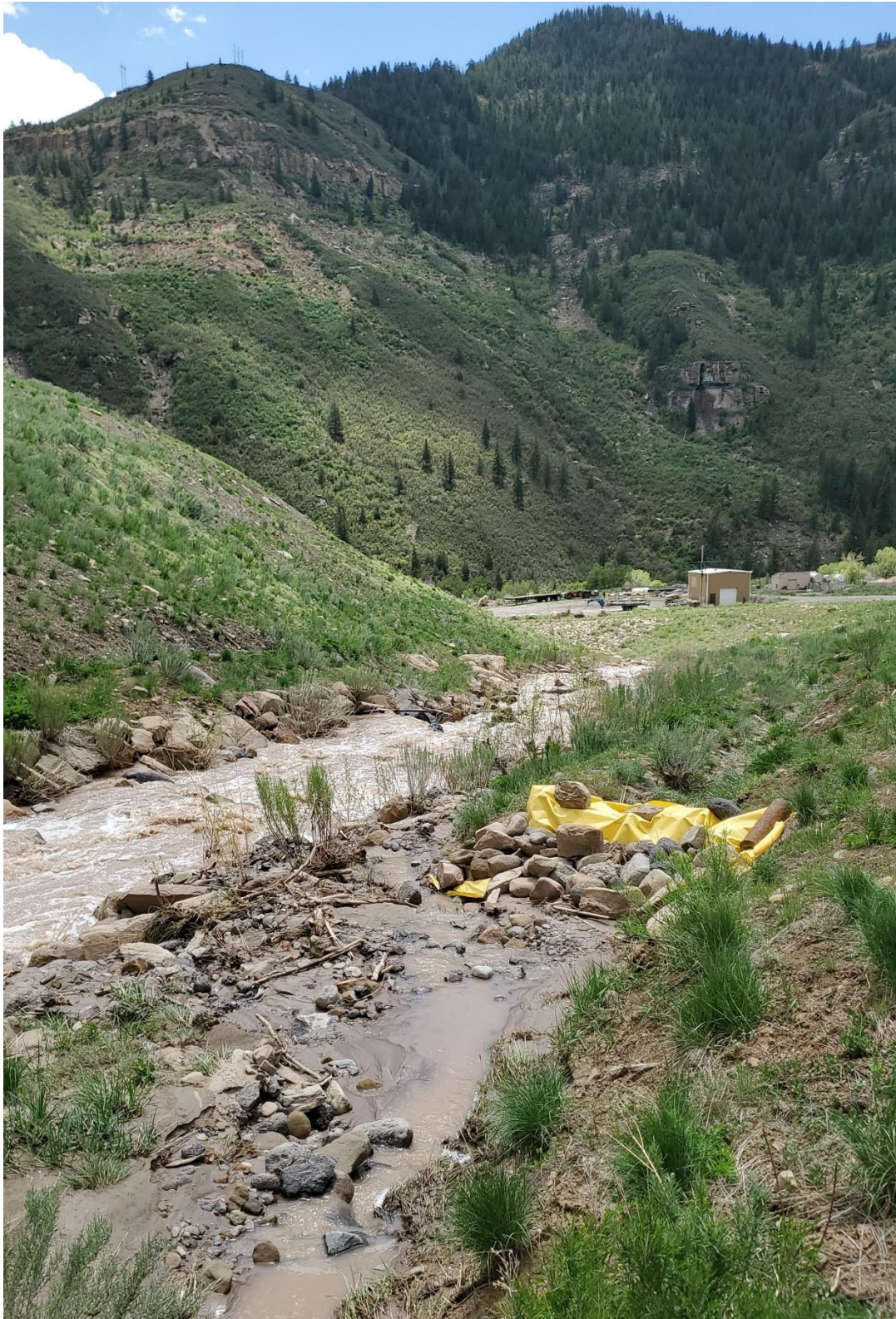
Figure 13: Dam used to divert water back into channel
