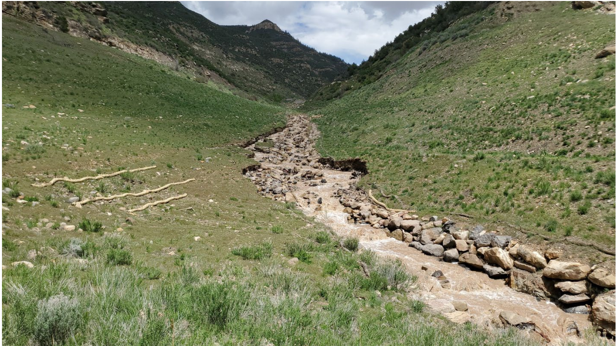
Figure 18: Fresh straw wattles placed in attempt to stabilize slope below Ditch T-1
