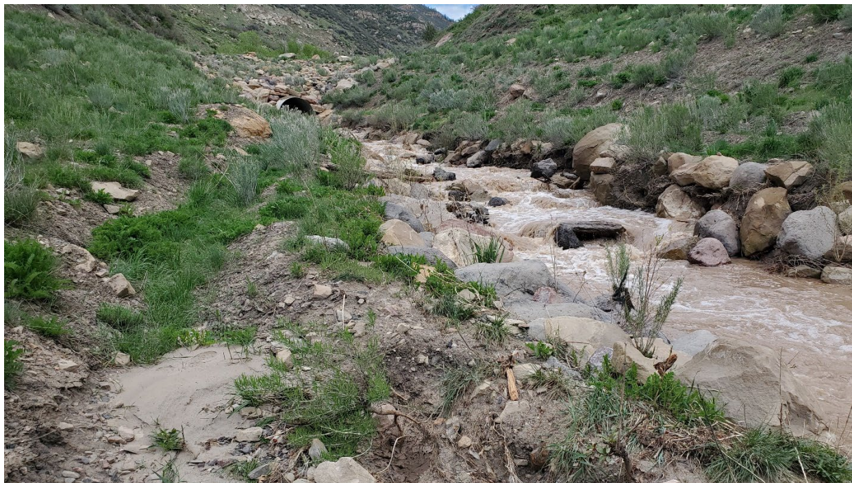
Figure 9: Point where Elk Creek first breached Ditch T-1, below outlet of first section of Elk Creek culvert
