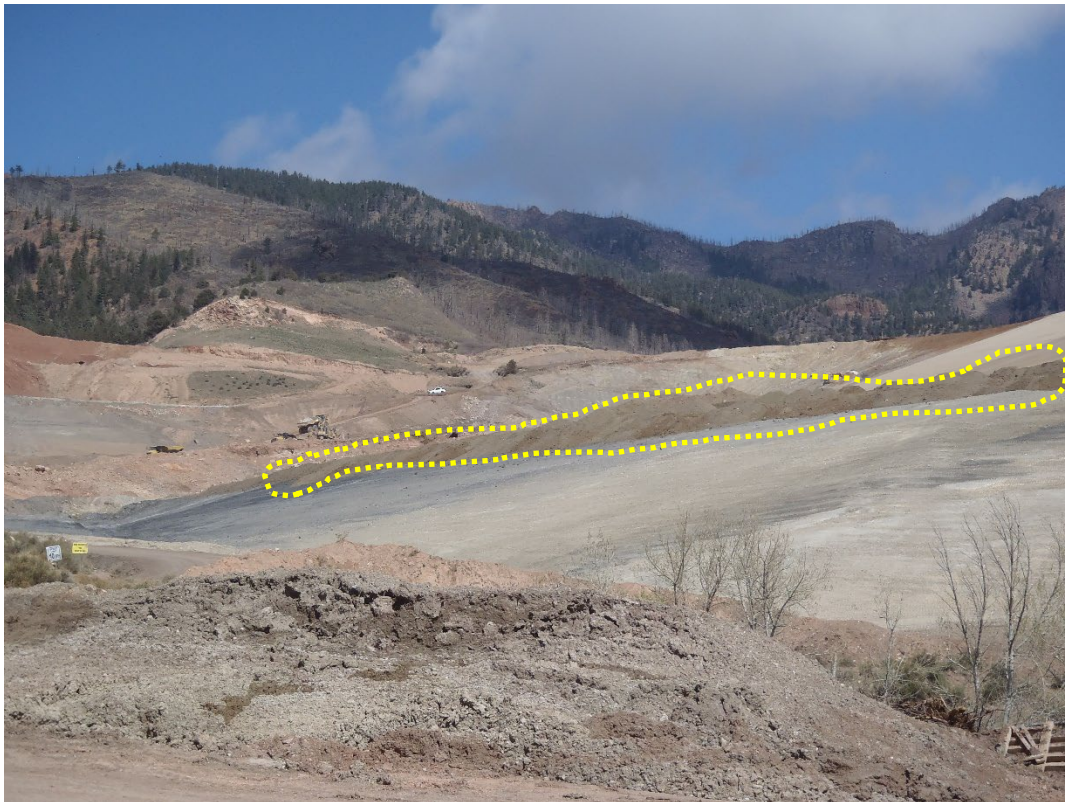
Photo 1. Nearly final grade in former shop area – topsoil (circled) placed at crest (looking NW).
