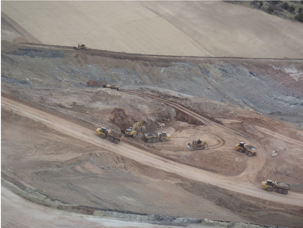
Photo 4. Material excavation from north (private area) borrow area (looking NE from above the slide area).
