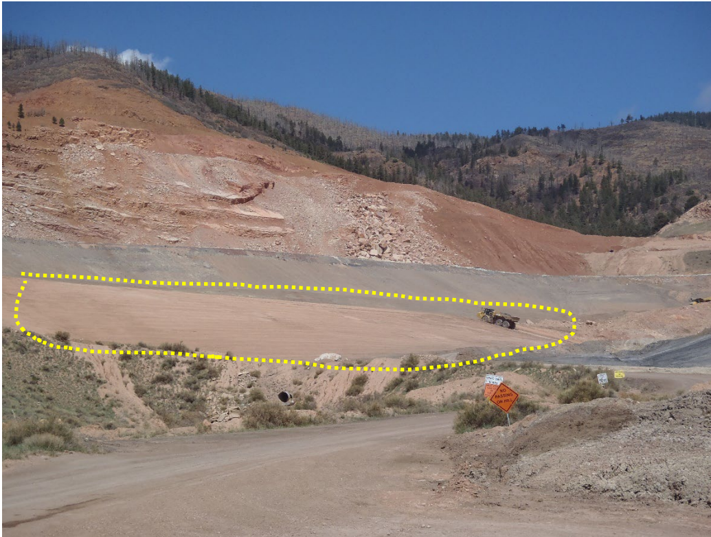
Photo 2. Recently graded lower slope between haul road and lowest bench (looking west).
