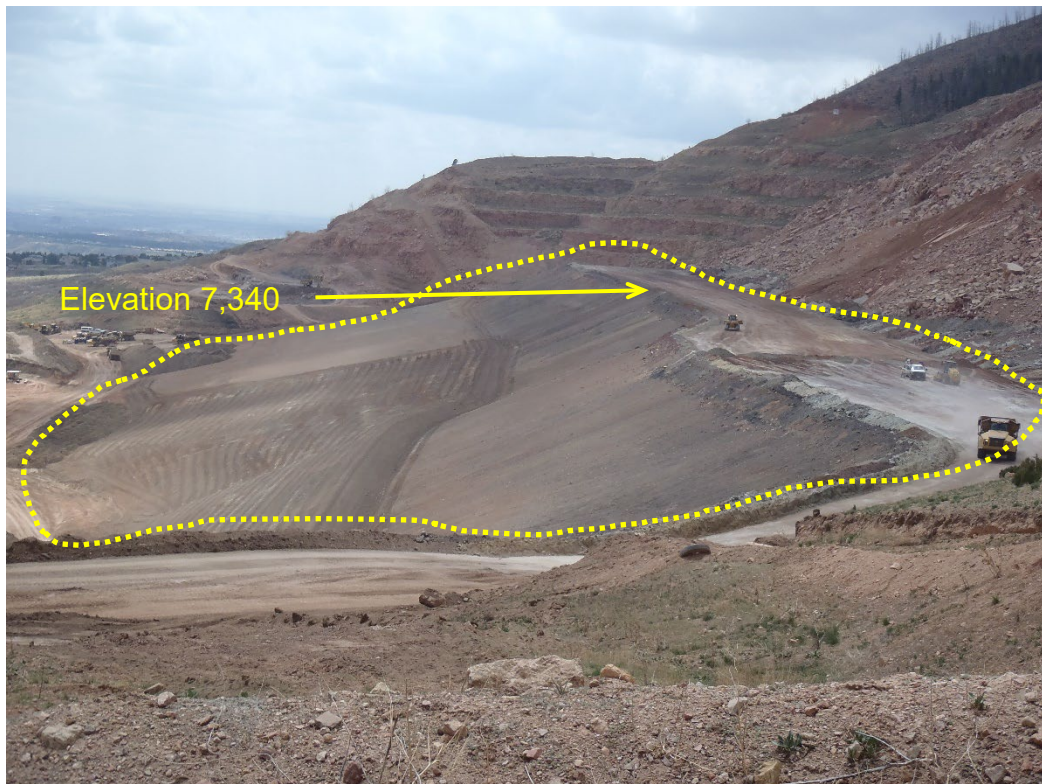
Photo 3. Placed and compacted buttress material (circled, looking south).
