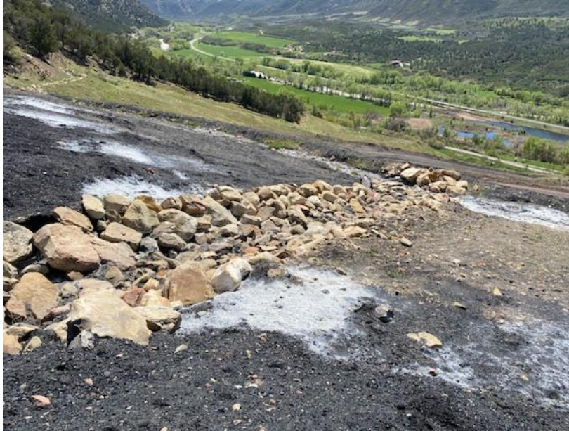
Photo 5: The riprap channel near the top of Gob Pile #2.
