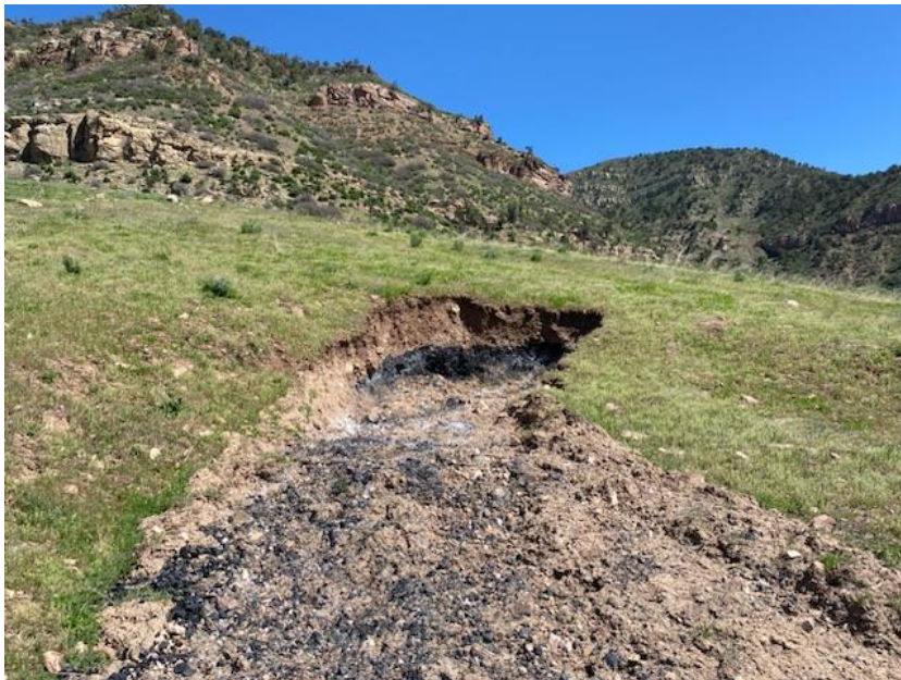
Photo 4: Sloughed material on Gob Pile #4.
