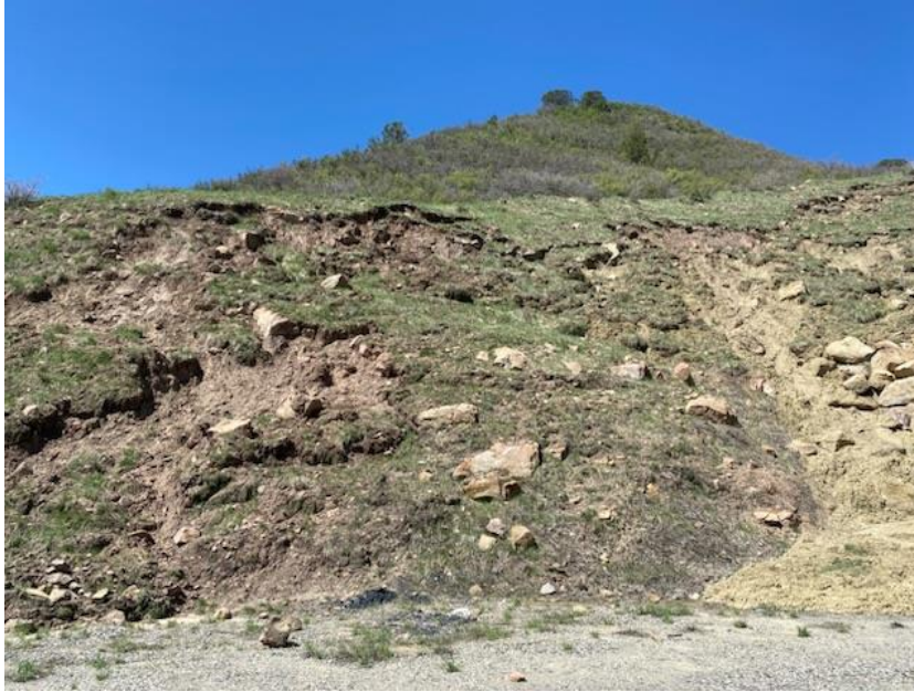
Photo 9: Slide on the southwest side of the B Portal bench
