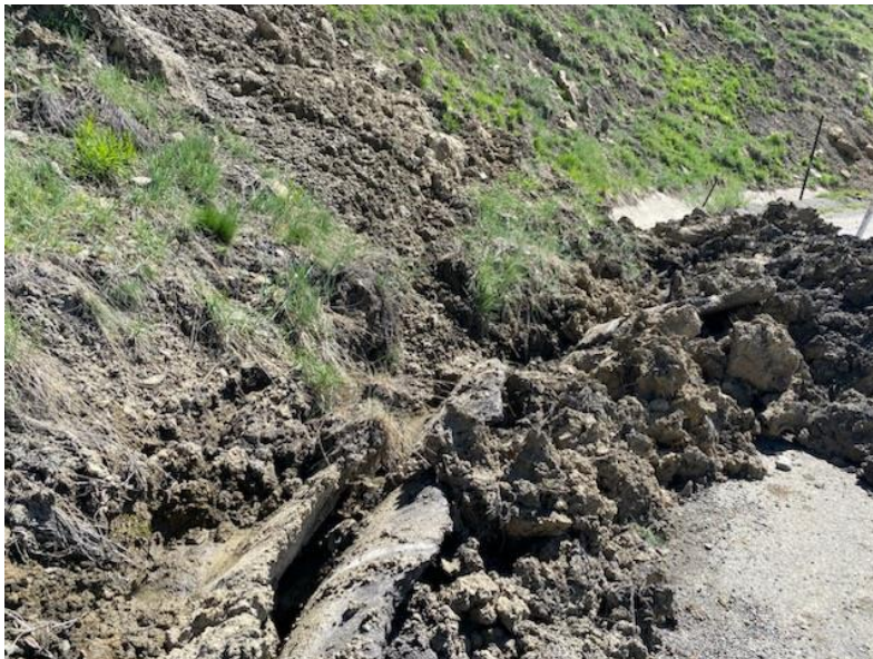
Photo 8: Temporary drainage cut through Curve 10 slide
