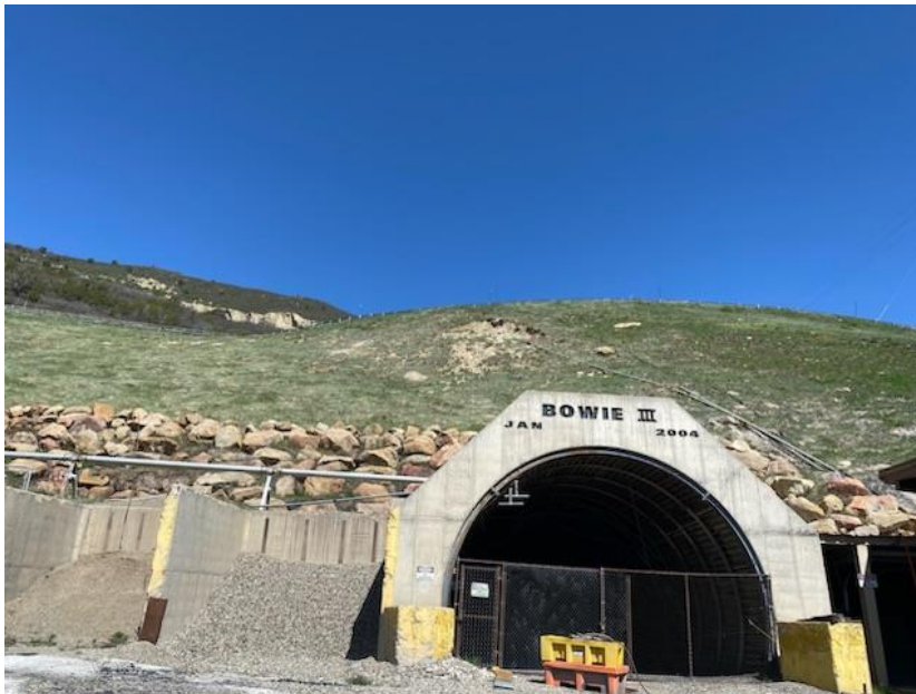
Photo 10: Minor slide above B portal
