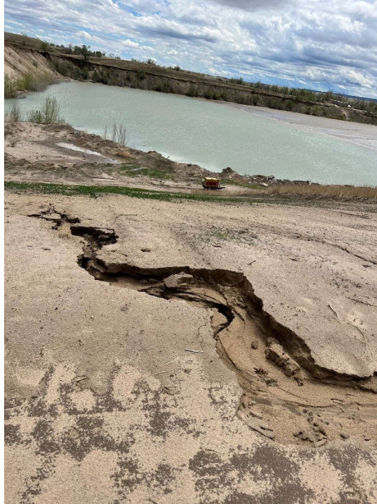
Photo 1. Fresh erosion gully near east end of buttress
