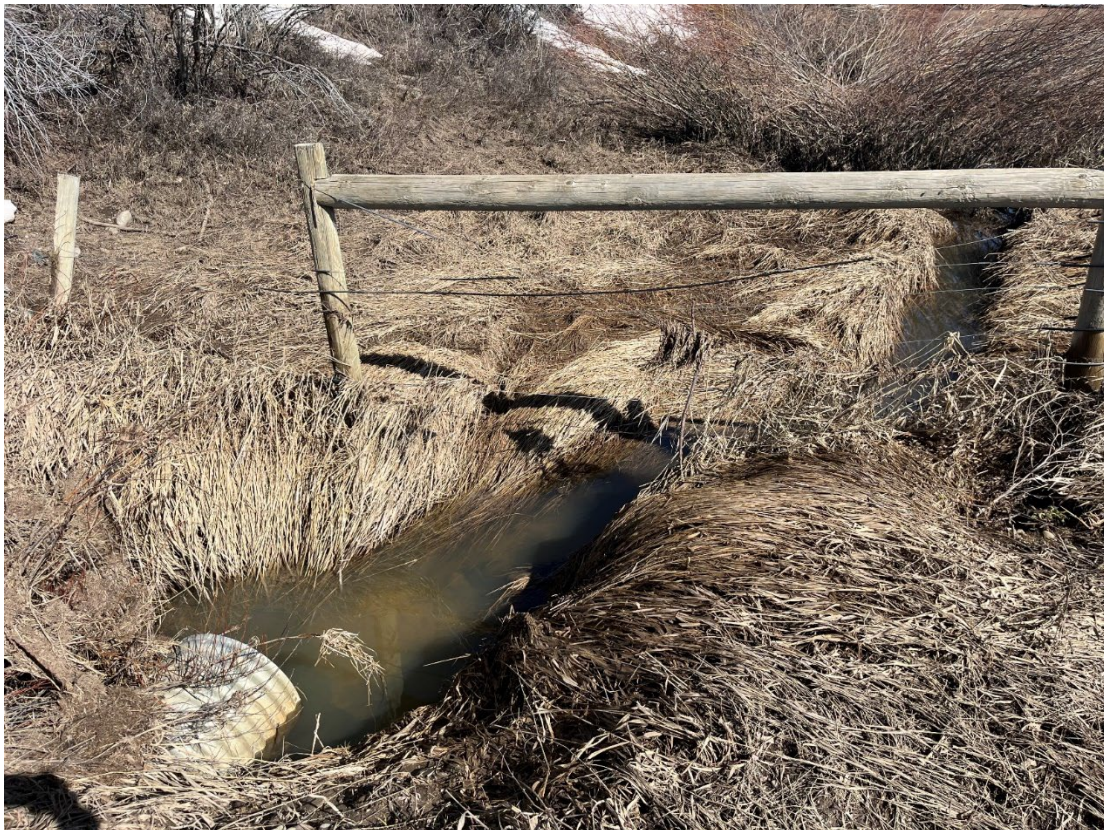
Photo 4: Culvert located to the north, just before the mine sign, carries water under the road to Cottonwood Gulch. Culvert was clean and functioning properly.
