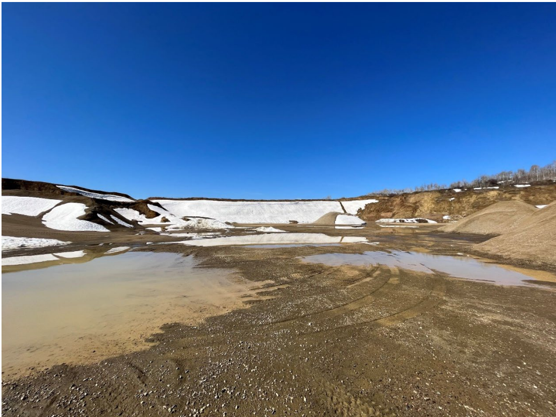
Photo 14: View south of various stockpiles. Topsoil is stored above this slope to the west.
