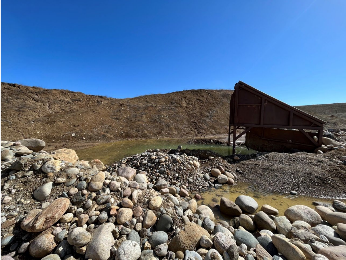
Photo 13: Area behind grizzly bars. Various stockpiles appear to be impounding several inches of water, blocking its flow to the approved drainage path of the site. See above problem citation.
