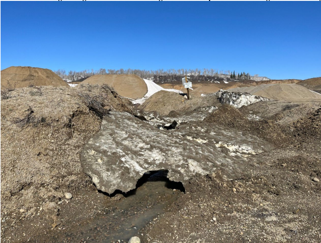
Photo 8: View north of sediment pond and break in the dam which is allowing water to flow into the ditch along CR62. See above problem citation.
