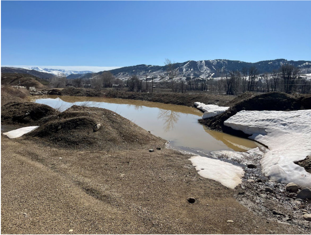
Photo 9: View east of the sediment pond to which all site surface water drains.
