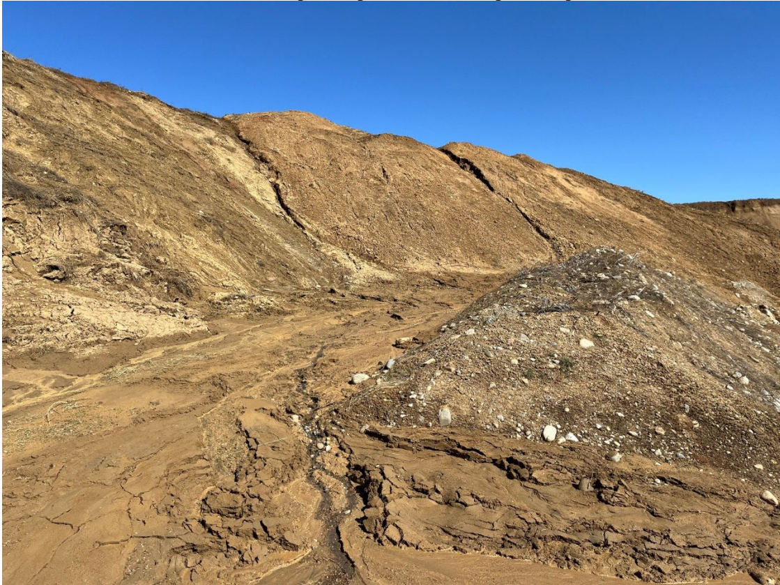
Photo 16: View northwest of deeply incised erosional features seen on stockpile.
