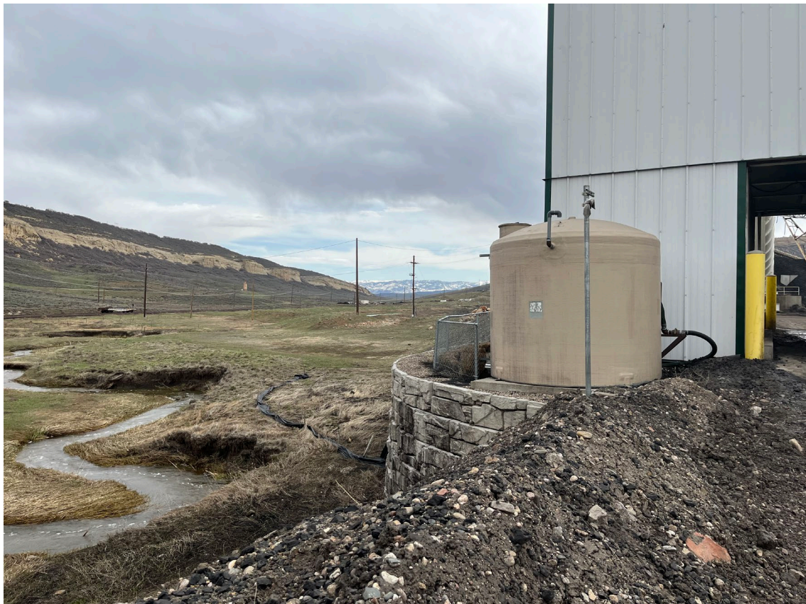
Photo 2: View NE of the back of the stoker coal loadout facility, Foidel Creek is directly below. A silt fence has been installed to protect Foidel Creek from sediment / runoff from this building.
