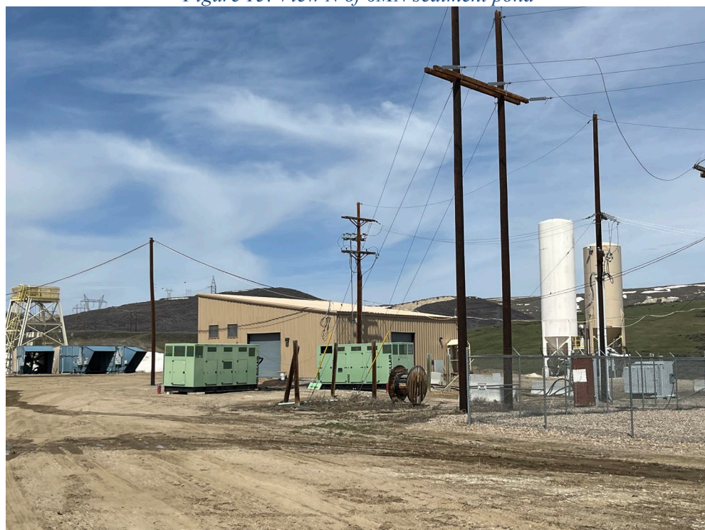
Figure 16: View N of 6MN facilities including 6MN intake shaft, emergency escape, rock dust containment, and electrical substation
