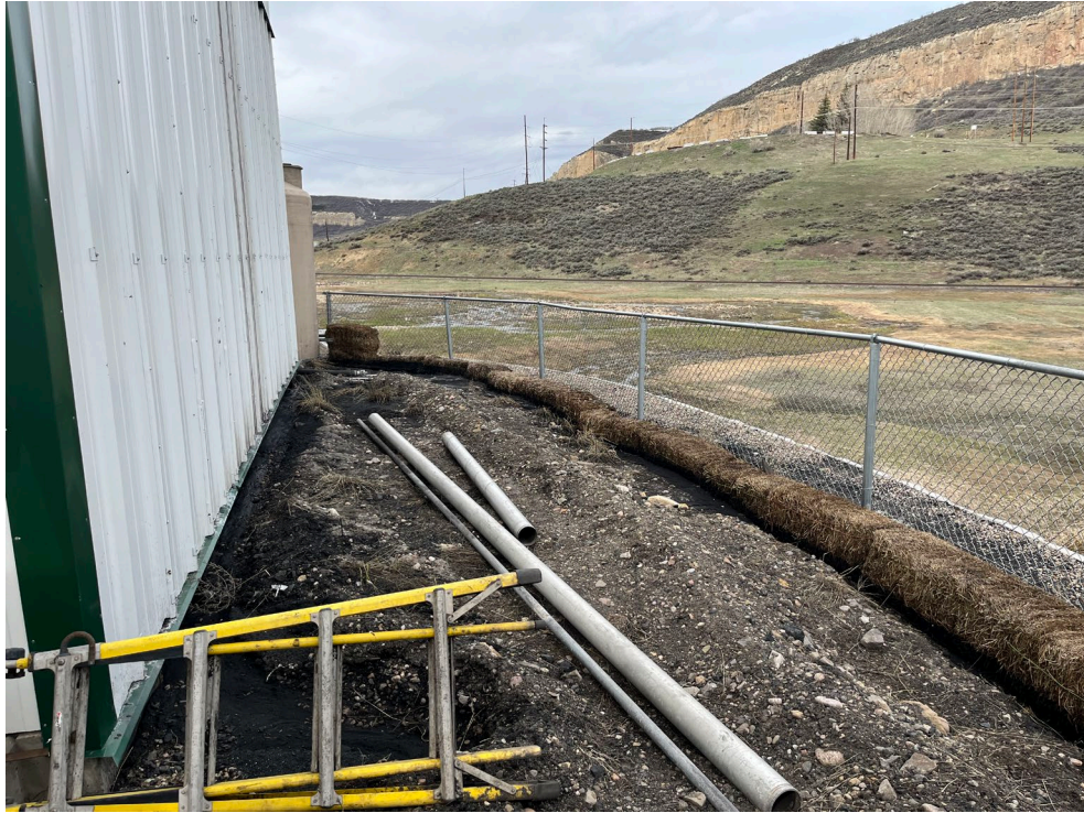
Photo 3: View S, behind stoker coal loadout building which shows the straw bales put in place to slow the drainage of water from the stoker loadout building to Foidel Creek below.
