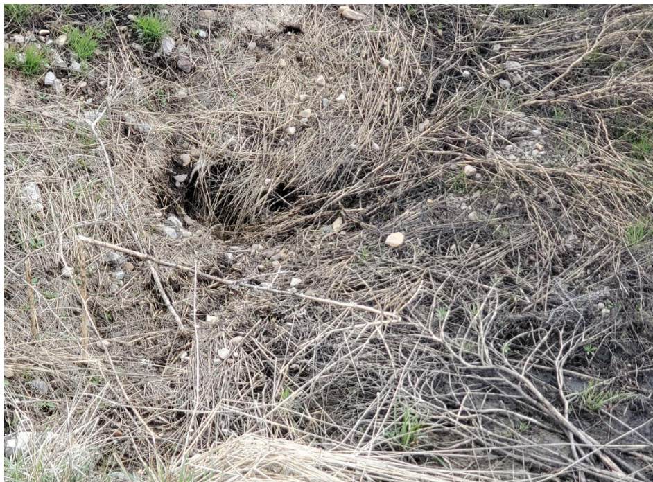
Photo 7: Plugged culvert near the Nitrogen Plant. View to the northeast
