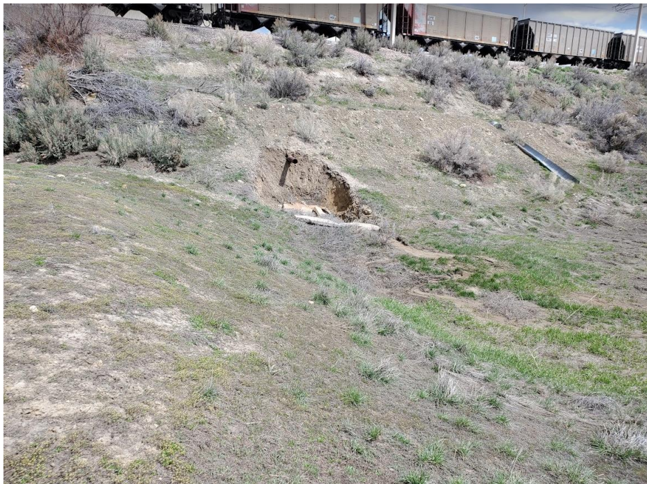
Photo 6: Erosion scar on Rail Loop Pond. View to the north.
