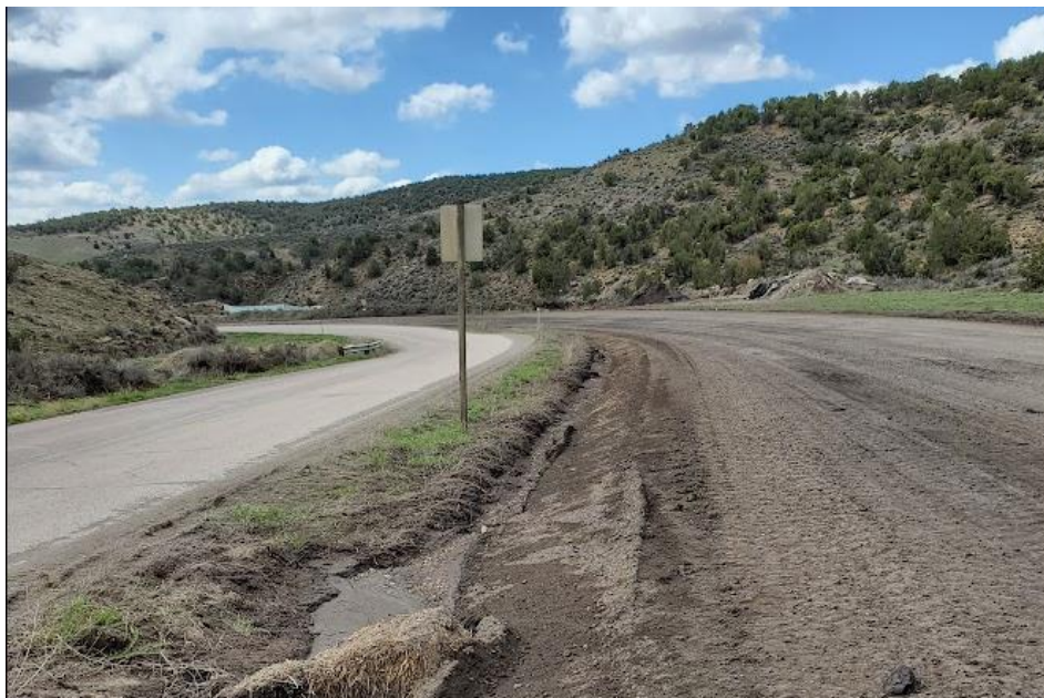
Photo 9: View to the south. Ditch that has been pulled along haul road
