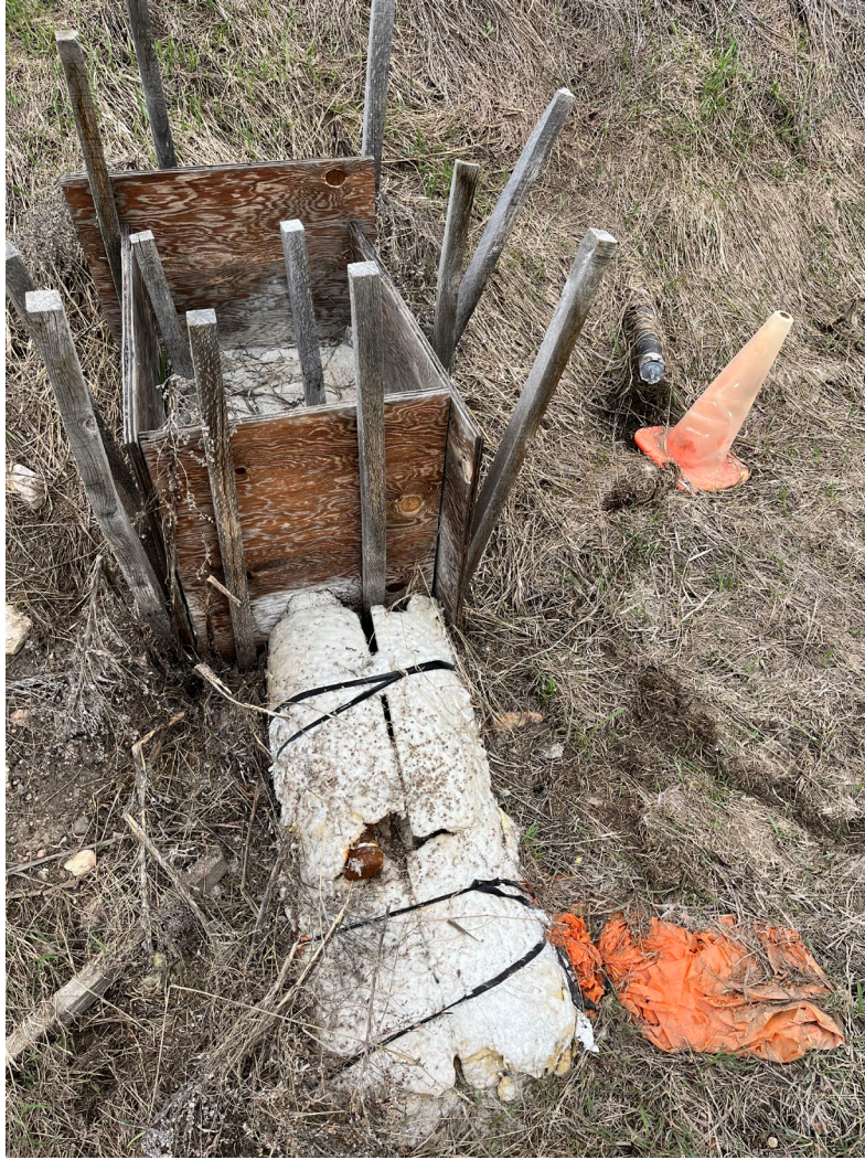
Photo 14: Leaky pipe as noted in previous inspection reports. Efforts have been made to protect pipe from future blowouts.
