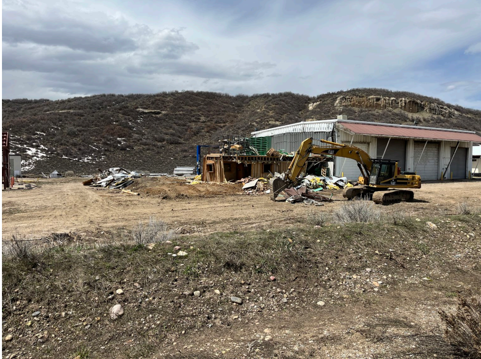
Photo 6: View W of a recently collapsed part of the vehicle maintenance shop, caused by the winter seasons heavy snowfall. Cleanup is currently underway.
