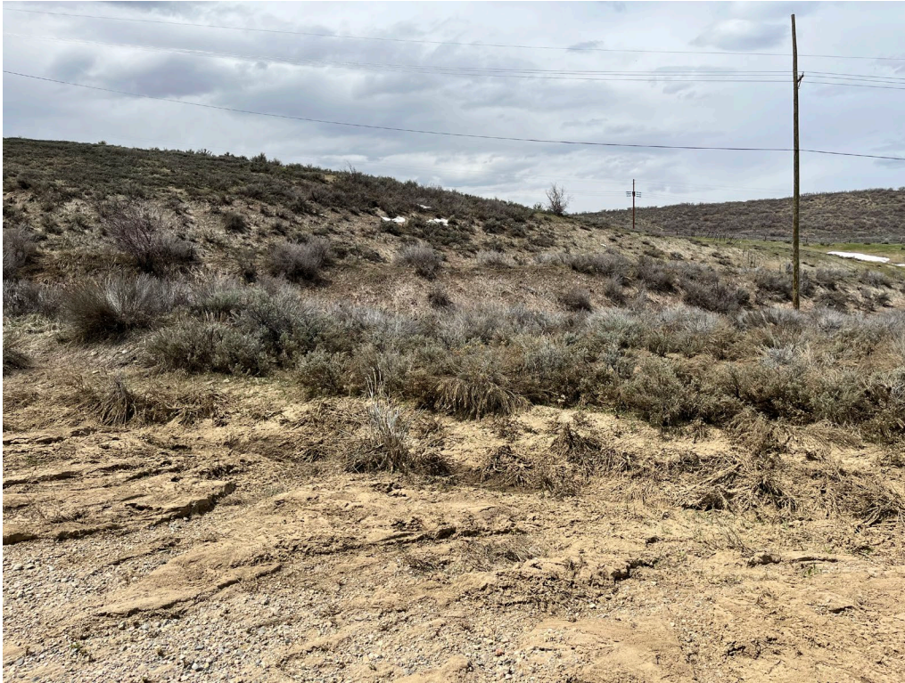
Photo 8: View W from Road B, recent flooding overtopped this road, causing small amounts of erosional damage to the road. See maintenance items.
