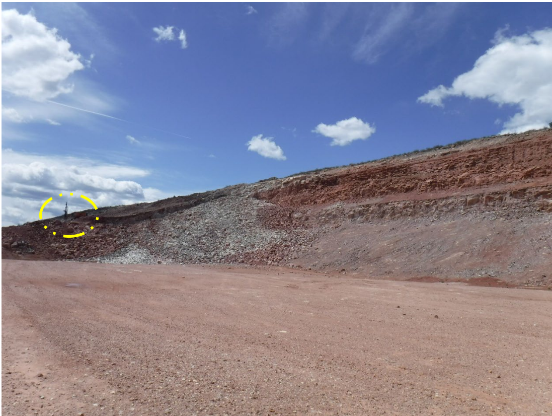
Photo 6: Blasted rock material, drill rig circled in yellow
