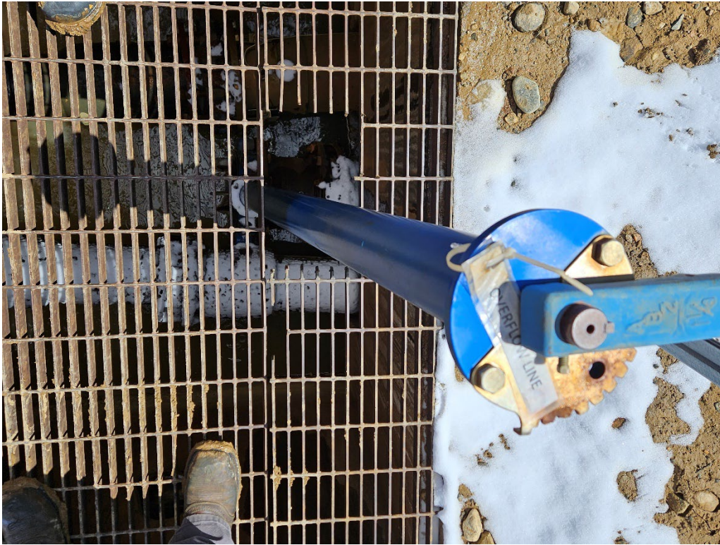
View of the 3-Dam backup seepwater line discharge valve
