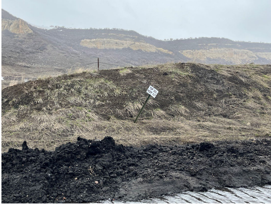
Photo 2: Topsoil piles throughout the site are appropriately marked and undisturbed by the winter season's snow plowing. Piles will be reseeded later in the spring.
