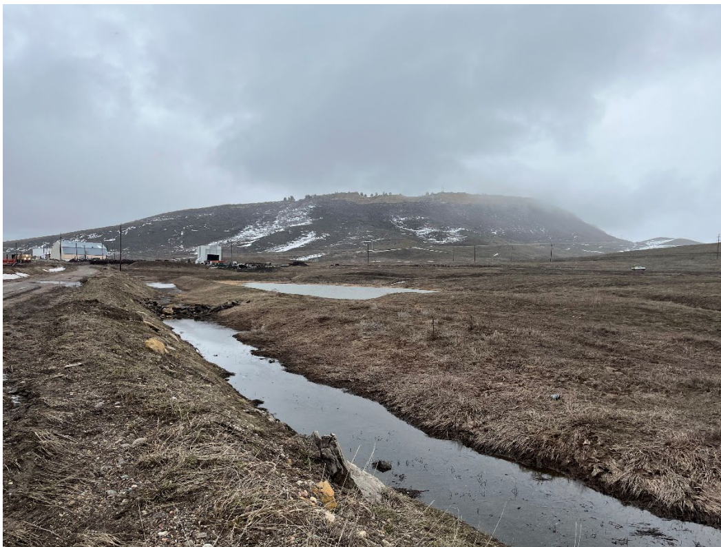
Photo 10: View northeast of Pond F. Ditch is functioning properly to divert the large amounts of snowmelt flooding into Pond F.
