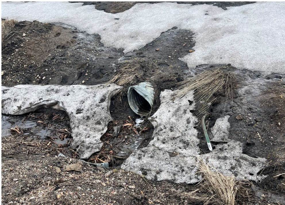
Photo 8: Culvert which discharges Pond C, freely flowing.
