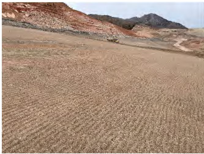
6. Slope at final grade leading up to first bench
