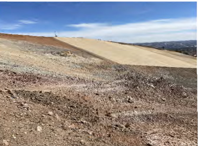
2. Erosion blanket on slope in North Borrow Area.
