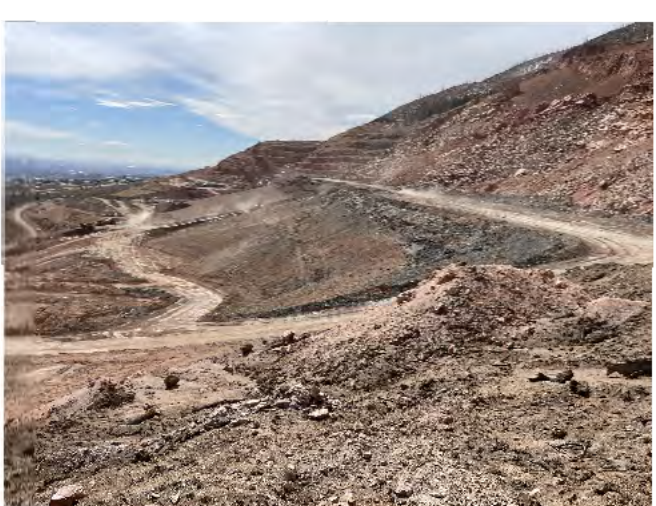
3. View of compaction area and first bench.
