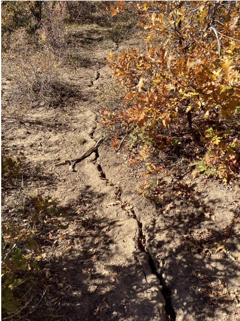
Figure 4: One of the downhill, parallel cracks observed at Location 3, south of the across road on Traverse C-C'.
