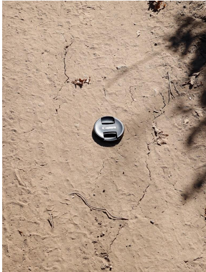
Figure 2: East-Southeast view of small subsidence crack diagonal across road on Traverse C-C' near Location 2.
