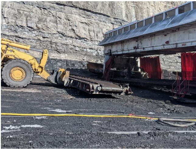
Highwall mining operation at South Taylor Pit.
