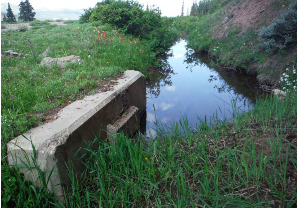
5ST1484.1, Old Colorado State Highway 91 Loop (F1) and concrete culvert (F4) at front, view to west.
