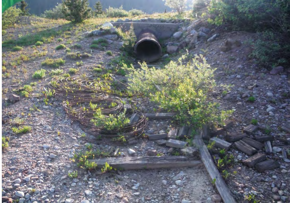
5ST1485.1, Fremont Ditch (F1) and concrete culvert (F3), view to east.
