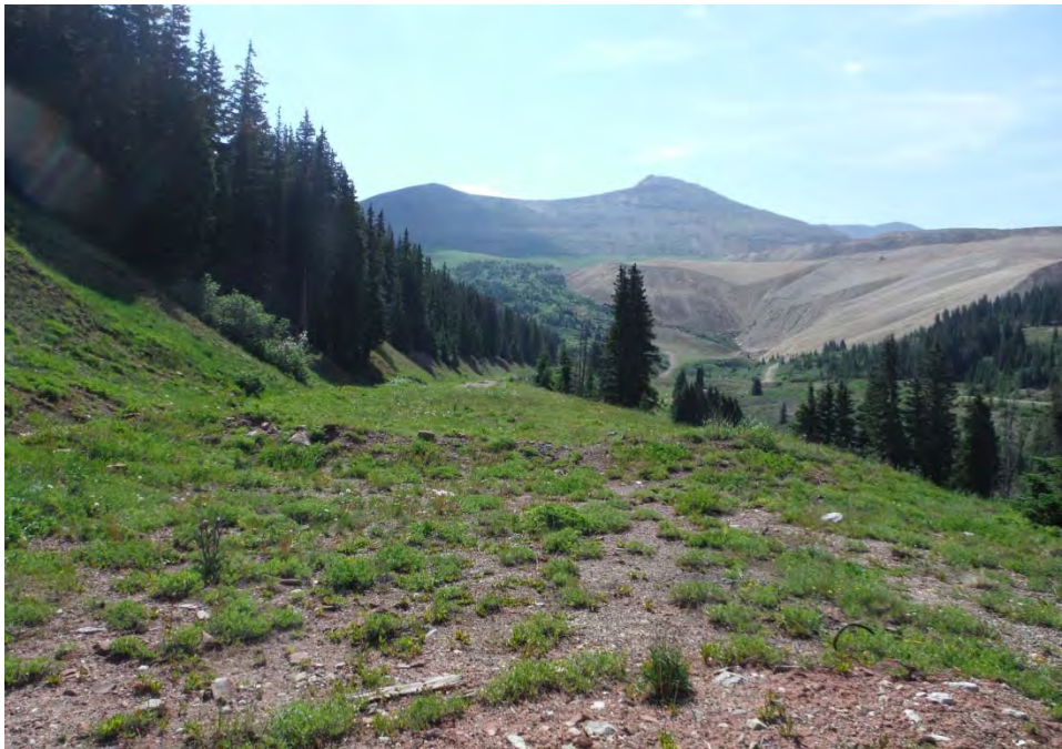
5ST1484.1, Old Colorado State Highway 91 Loop, disintegrating pavement on the roadbed (F1), at western project area boundary, view to east.
