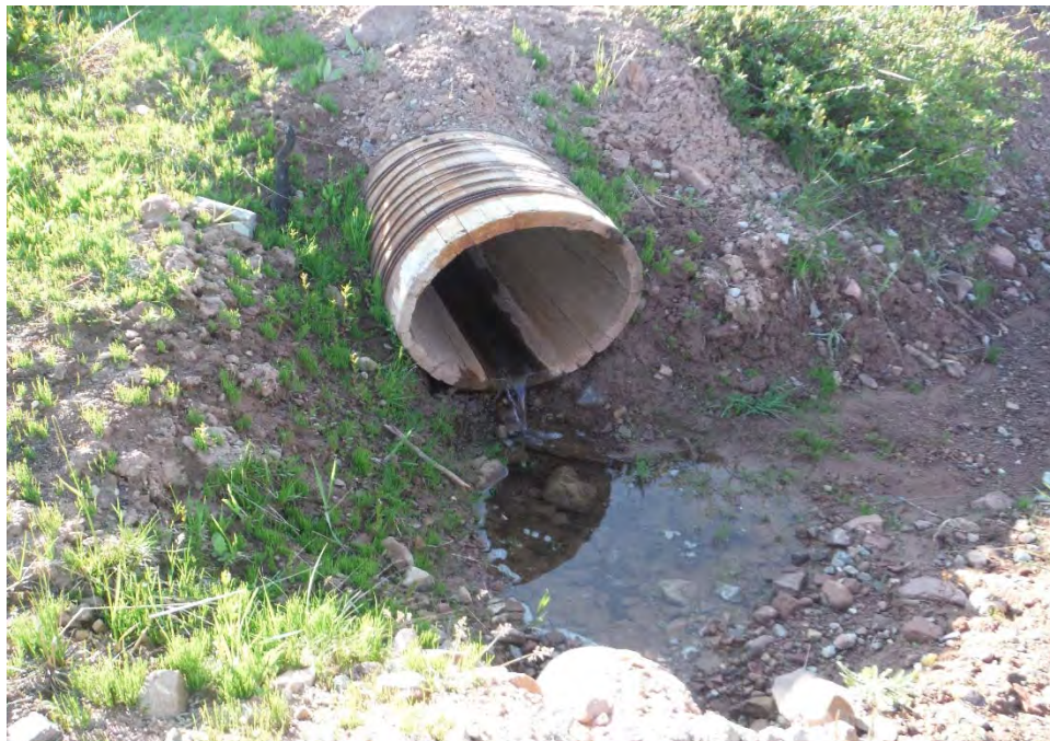
5ST1486.1, water diversion pipeline (F3), view to south.
