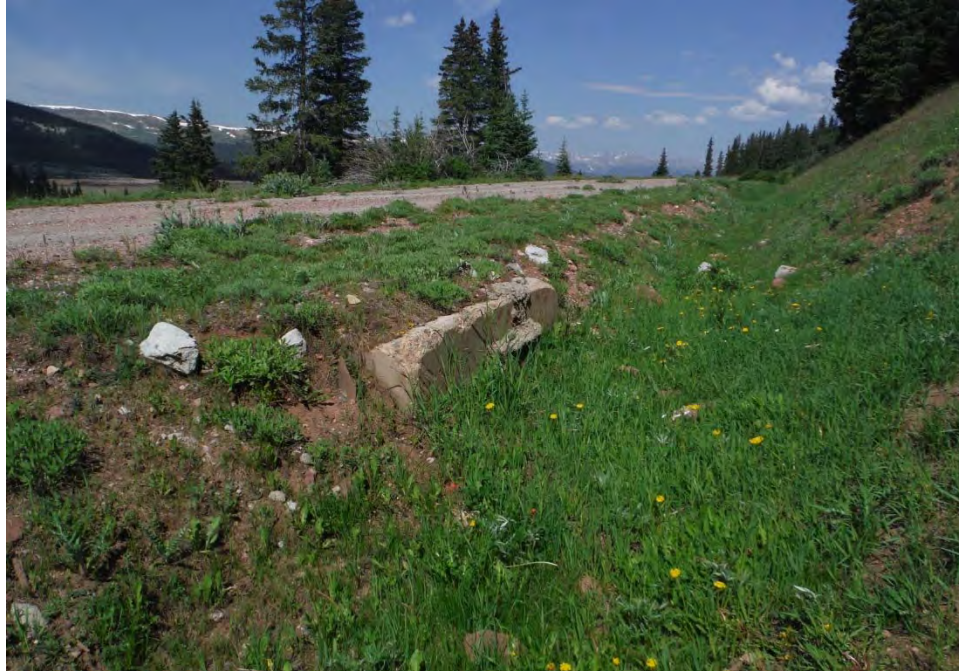
5ST1484.1, Old Colorado State Highway 91 Loop (F1) and concrete culvert (F3) at center, view to southwest.
