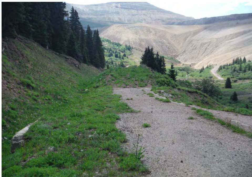
Site 5ST1484.1, Old Colorado State Highway 91 Loop (F1) and concrete culvert (F2) on left, view to east.
