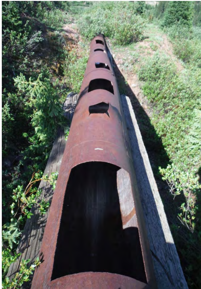
5ST1486.1, water diversion flume (F2), view to southwest.
