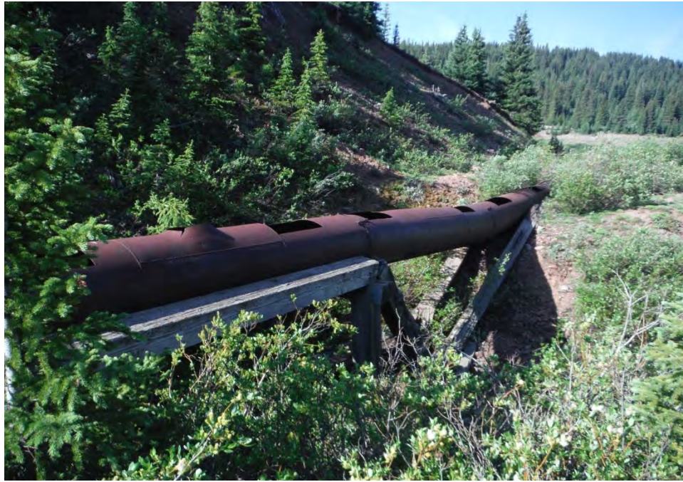
5ST1486.1, water diversion flume (F2), view to south.
