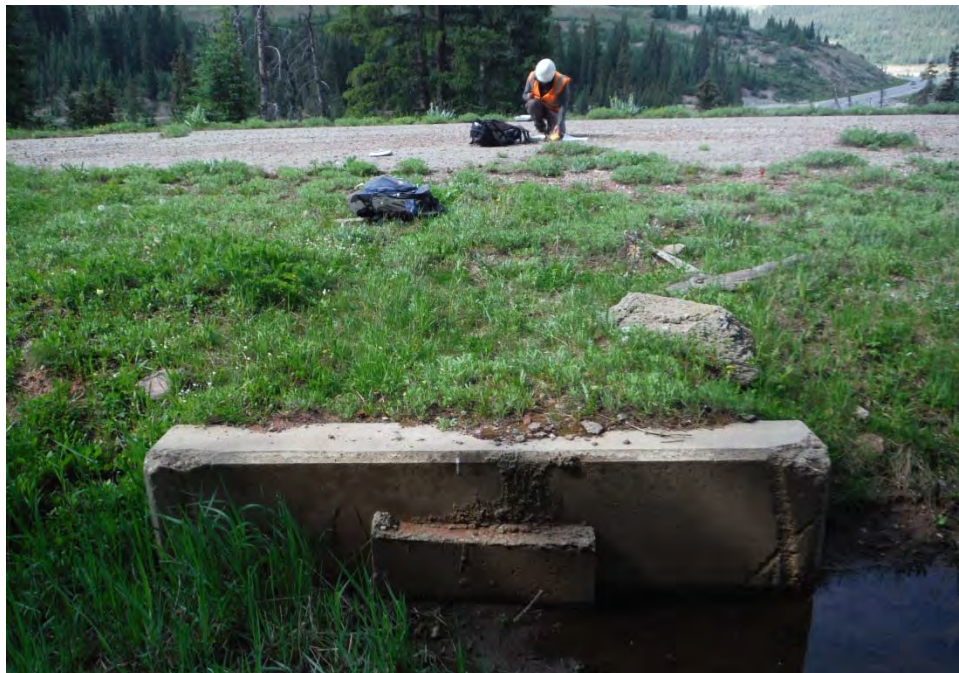
5ST1484.1, Old Colorado State Highway 91 Loop (F1) and concrete culvert (F4) at front, view to southwest.
