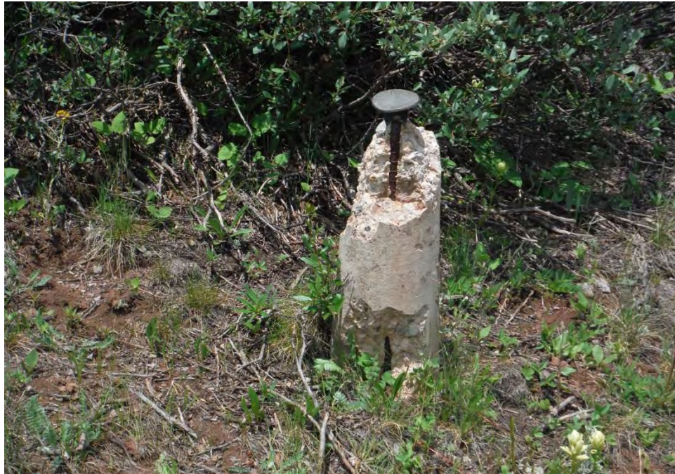
5ST1484.1, Old Colorado State Highway 91 Loop (F1) and State Highway Department right-of-way marker (F5), view to north.
