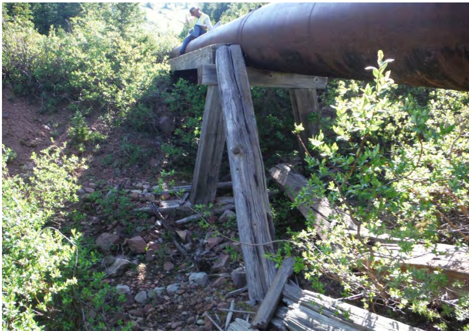
5ST1486.1, water diversion flume (F2), trestle supporting metal flume, view to northeast.
