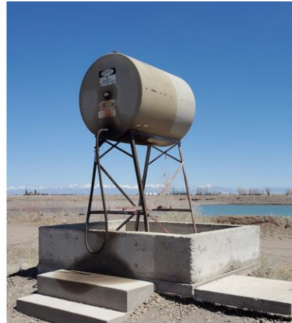
View to the east showing fuel tank along eastern boundary in concrete secondary containment.
