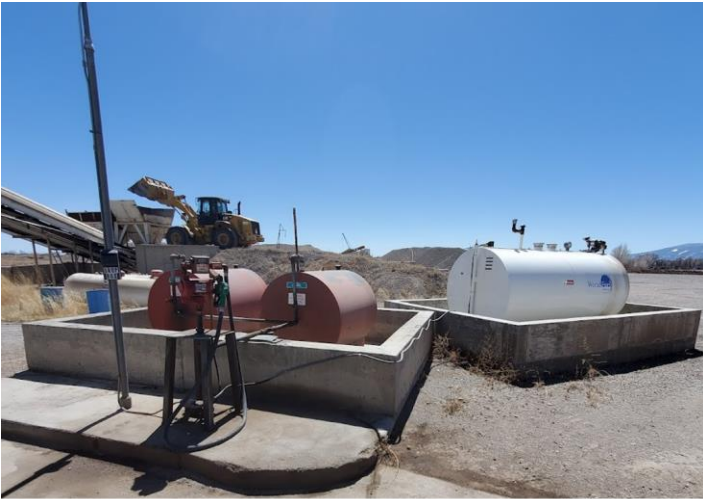
View to the south showing fuel tanks in secondary containment.
