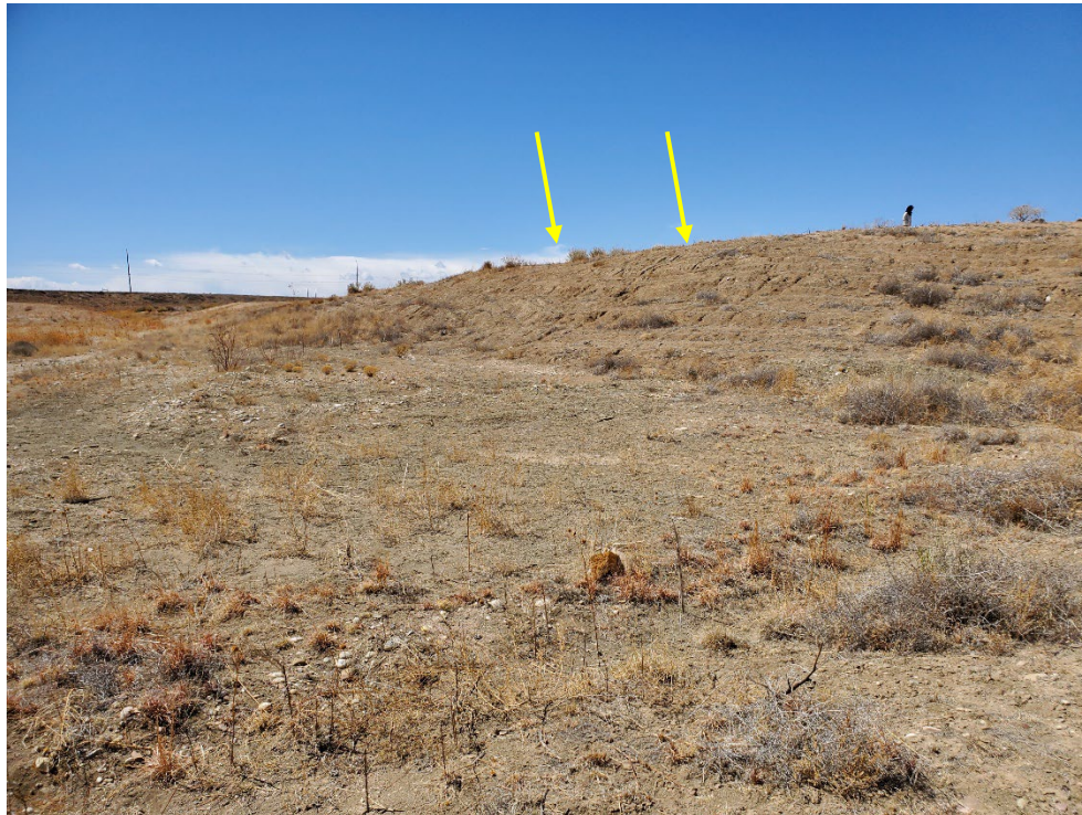
Photo 24: Standing on eroded berm in the north portion of Phase I, looking south-west across the reclaimed pit at the eastern face of the western slope. Yellow arrows point to slight rilling. This western slope has a greater quantity of stable vegetation growing than the eastern slopes.
