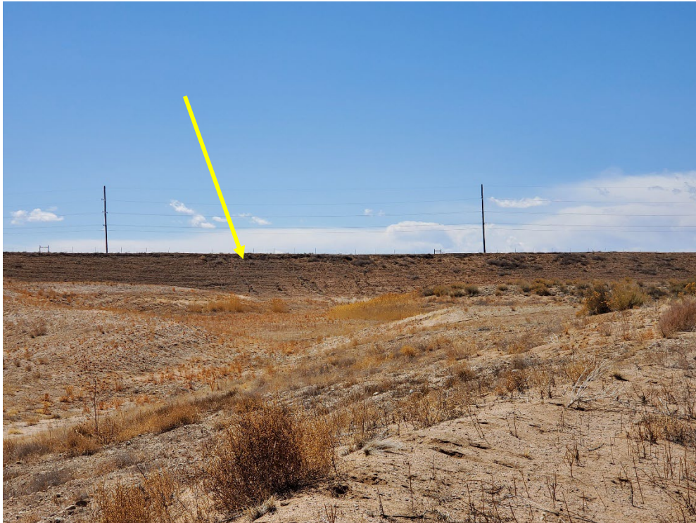
Photo 13: Standing on the western edge of the Phase 1 area, looking south at regraded slopes. The yellow arrow points to a slope that is the regraded highwall near the southern boarder from the 2020 Inspection Report. Some rilling was observed on this slope.
