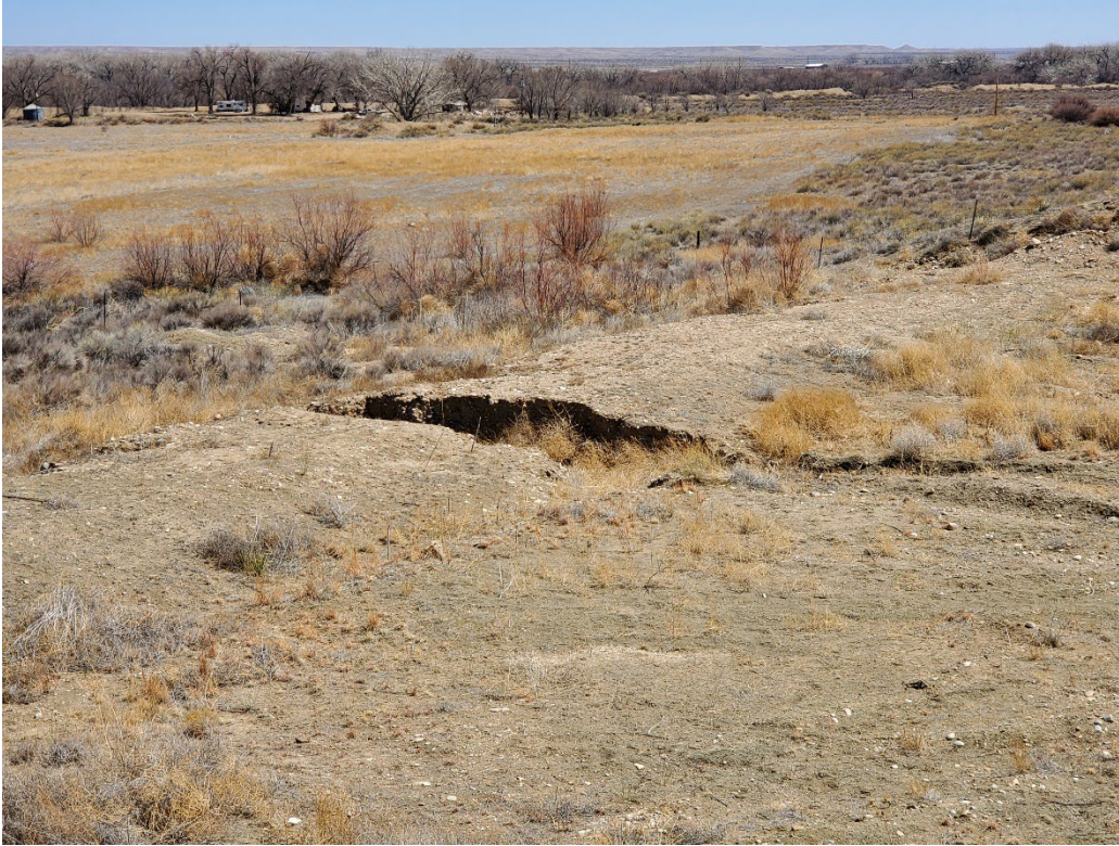
Photo 19: Looking north-east at the edge of the reclaimed Phase 1 area at an erosional feature in a bordering berm.
