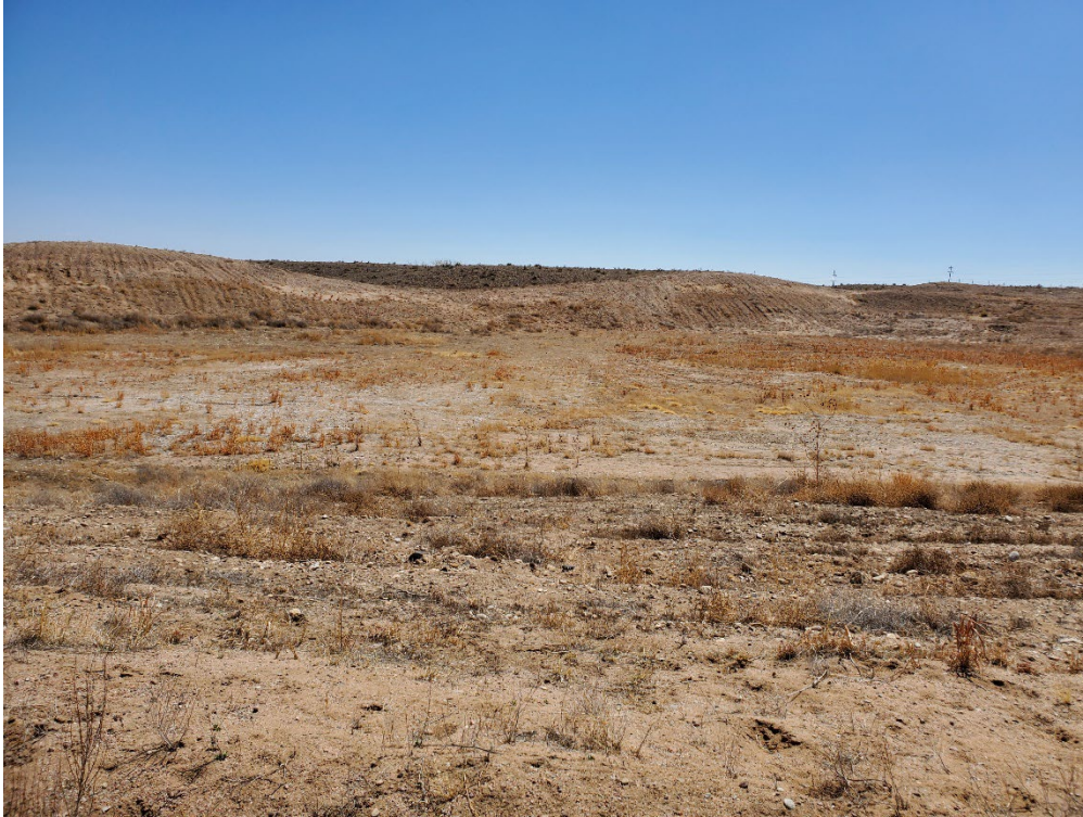
Photo 15: Standing on the western edge of the Phase 1 area, looking east across the seeded pit area and at regraded slopes. Rilling is seen on the west facing sides of the re-graded slopes.
