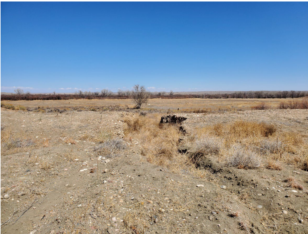
Photo 20: Standing in the Phase I reclaimed pit, looking north at the eroded berm and at the flood plain beyond it.
