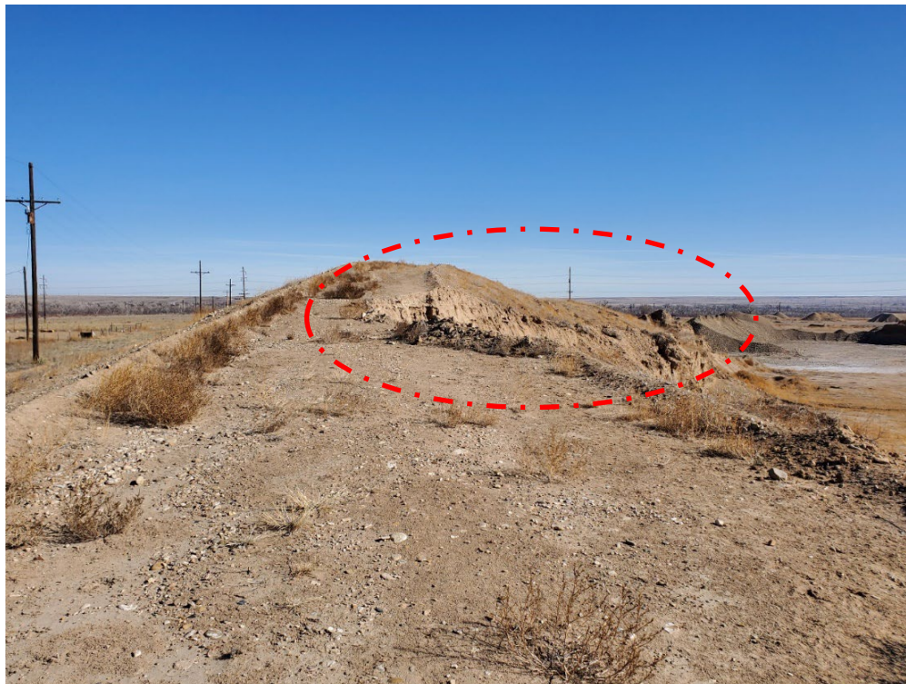
Photo 16: Looking east at the topsoil pile on site. This is located along the northern edge of the Phase 3 pit area. The area circled in the photo indicates where the topsoil pile has sustained damage from mining activities.
