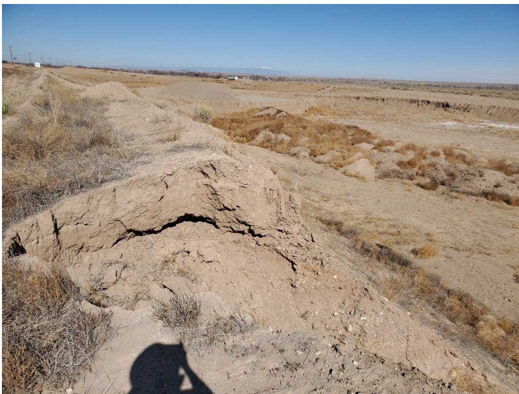
Photo 30: On top of the southern-most highwall in the Phase 2 area, looking at an erosional feature in the highwall.
