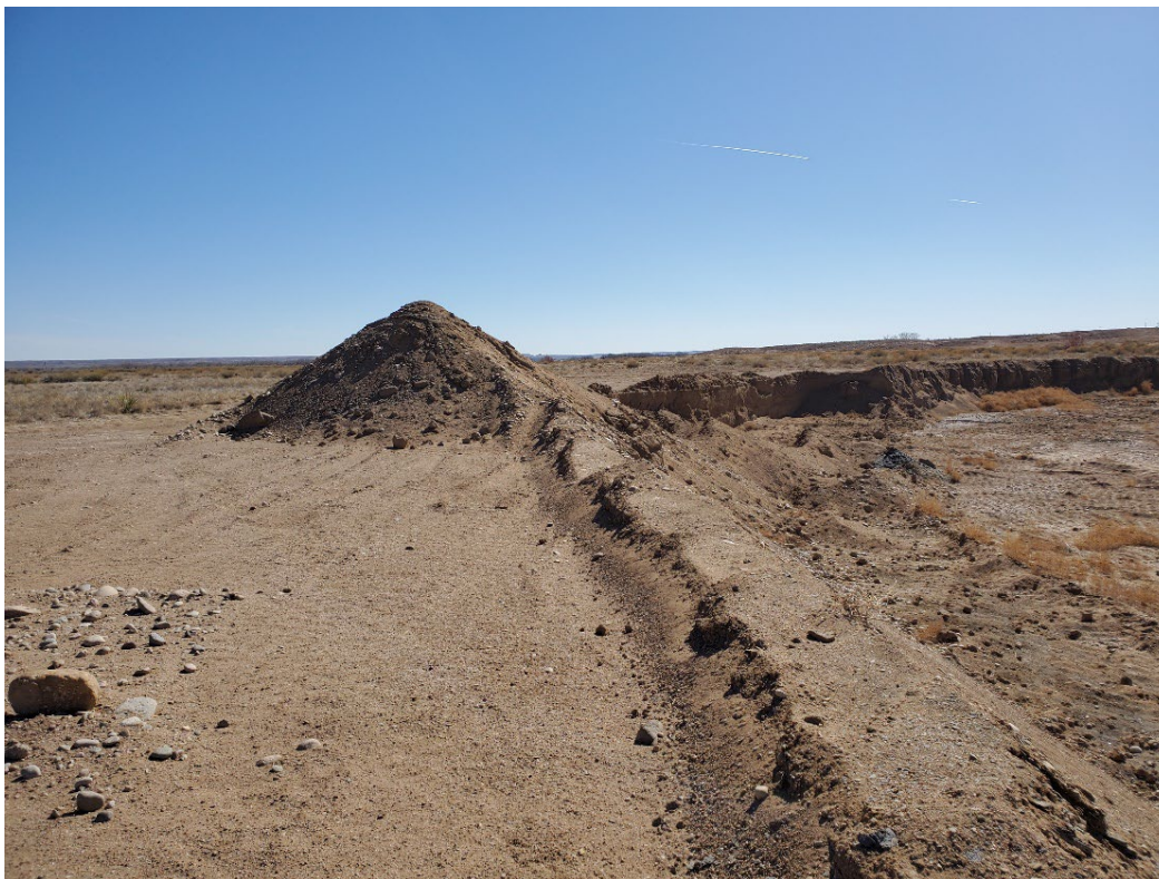
Photo 37: Looking east across the southern-most highwall in the Phase 2 area at excess material that may help with backfilling the highwalls.
