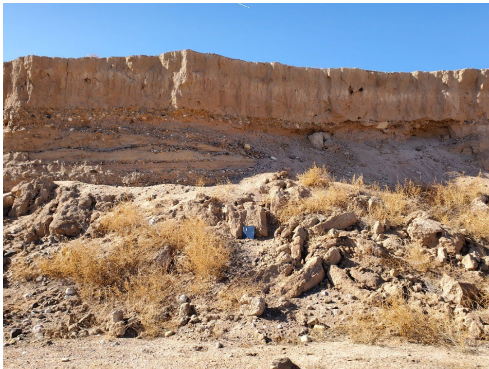
Photo 20: Looking West at maximum highwall height. Binder (11.5" x 10") for scale. Highwall is approximately 20' tall.
