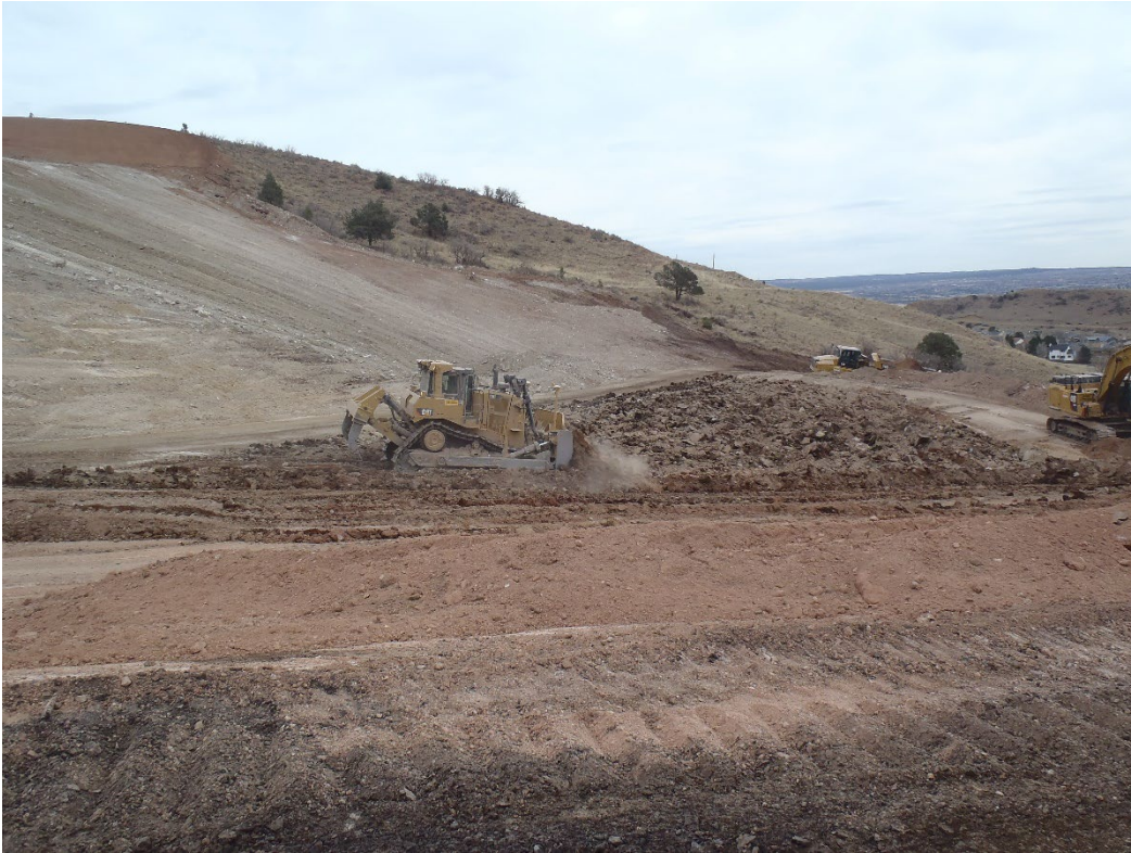
Photo 5. Full height of backfill placed (between dotted lines) to date (looking west from toe area).
