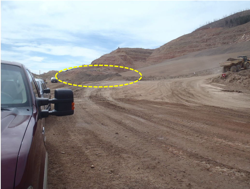
Photo 7. Topsoil ready for spreading on lower tier of backfill (looking south from backfill toe).
