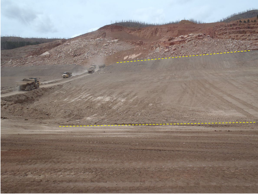
Photo 3. Full height of backfill placed (between dotted lines) to date (looking west from toe area).
