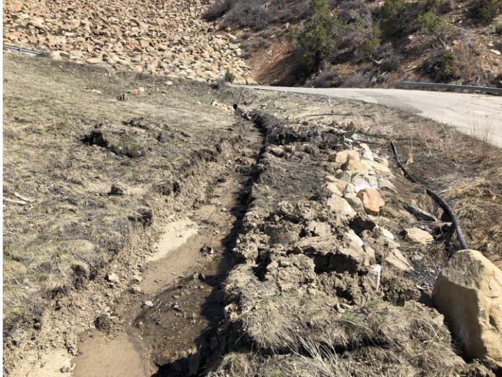
Temporary repair of Ditch B10 (Curve 8 in background)
