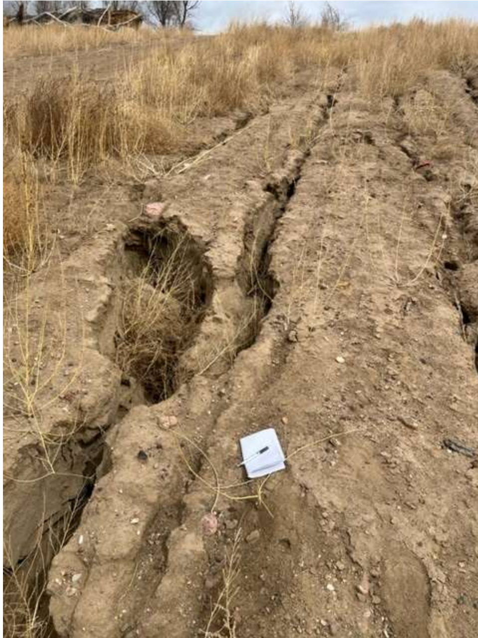
Photo 4. Representative image of erosion gullies near west end of buttress
