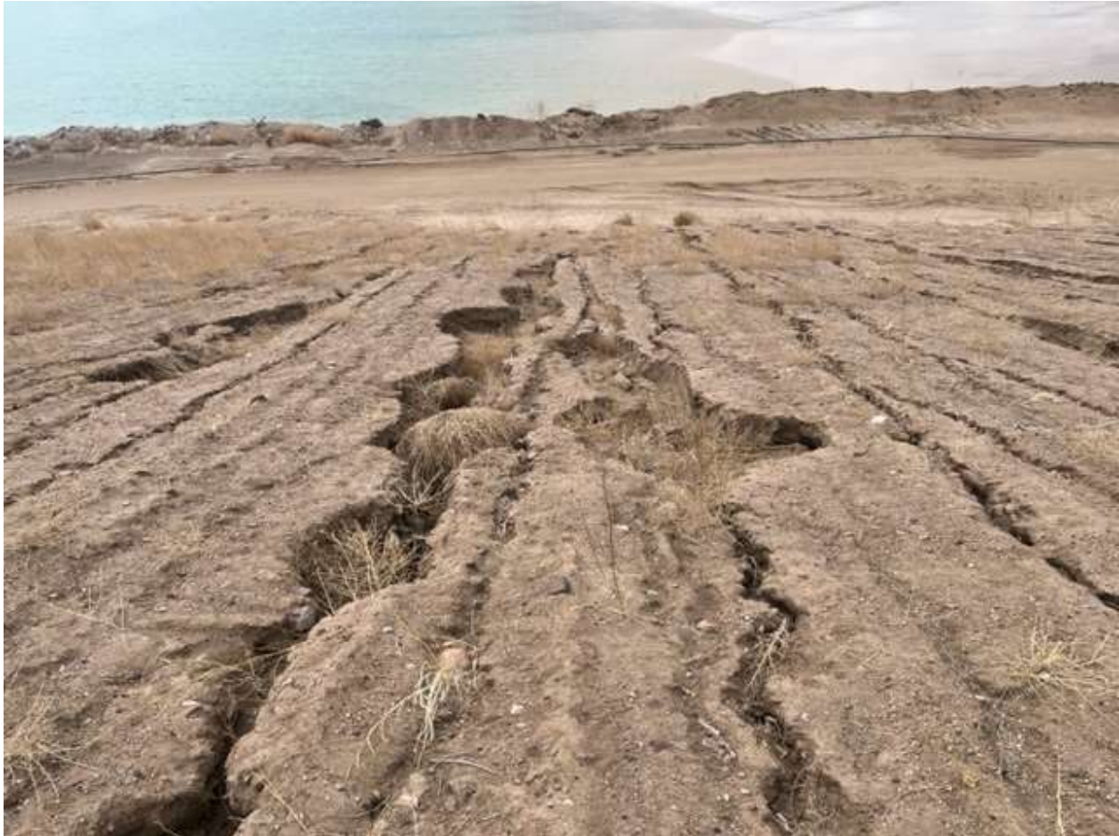
Photo 1. From the top of the buttress, looking down the slope, approximate 4 ft wide erosion gullies in central area of buttress are present.
