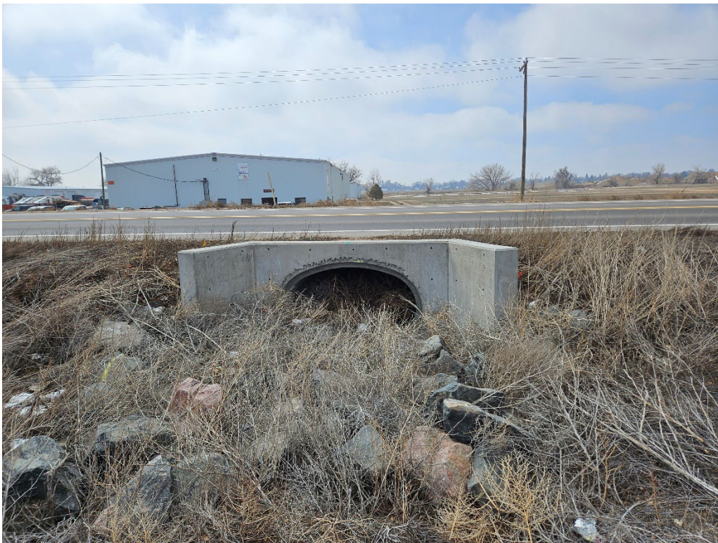
View of the culvert under 8 th Street in the southeast corner of the site to be used for dewatering
