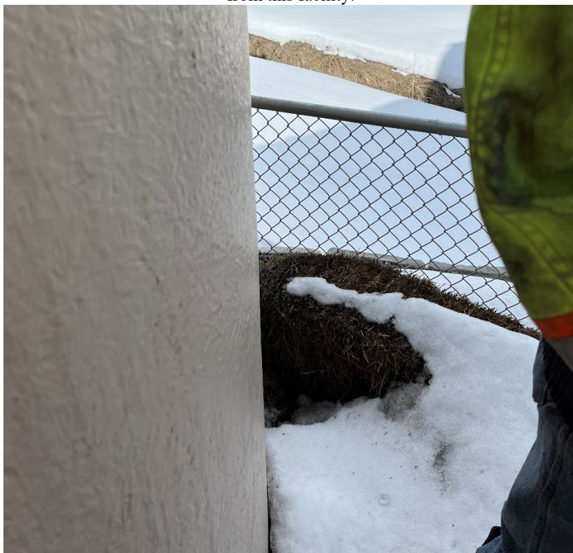
Photo 5: Straw bales placed upgradient of the three ditches located behind the coal stoker loadout building.
