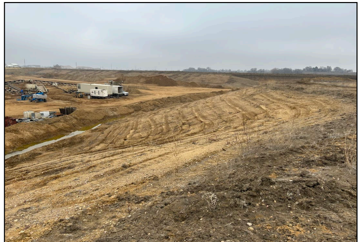
Photo 4 – Looking at representative area of re-sloped outer pit perimeter. Most of the north half of the pit perimeter has been re-sloped at this time.
